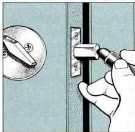
8 Test bolt for proper operation, then when satisfied, coat end of bolt with lipstick, close door and slide bolt onto jamb.
