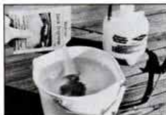
Mix one 6.4-ounce packet in 1 gallon of water. This will provide 150 sq. ft. of coverage.
