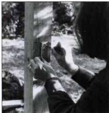
4 Mark position of metal fence brackets on the 4x4 posts. The galvanized brackets are used to join the 2x4 rails to the posts.
