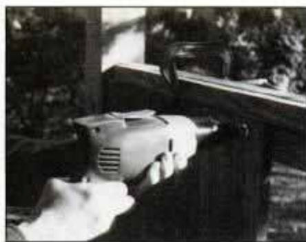
7 Fasten 1x6 fence boards to the 2x4 rails with 1½-in. screws. To keep boards even, butt them against cleat clamped in place.
