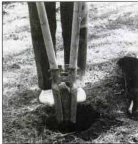
1 Dig fence post holes to about 30 in. deep with a post-hole digger. The hand tool is available from most rental equipment dealers.
