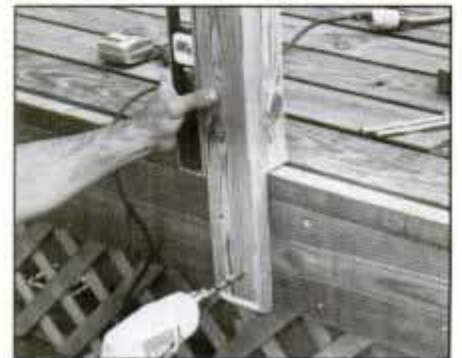
18 Hold notched post in place and plumb with level. Then bore pilot holes for lag-screws. Install lags and tighten securely.
