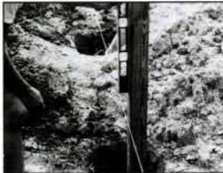
4 Slide each post into proper hole and align side with layout string. Plumb the post, then back-fill the hole with gravel.
