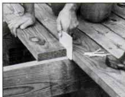
14 Maintain even spacing between decking boards by using wood spacer. Ends of boards must always fall over middle of joists.
