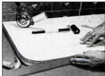
Start at one end and apply edge band. If you have to remove laminate, squirt lacquer thinner behind it to dissolve cement.
