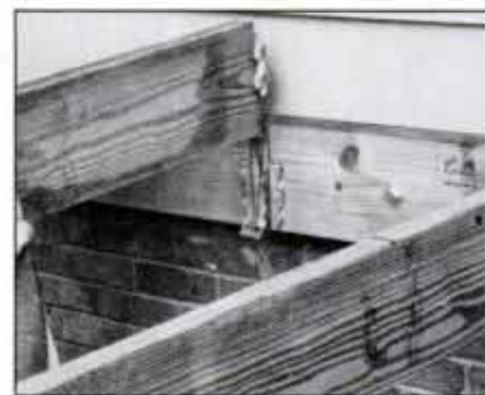
9 Attach joist hangers to ledger boards using nails provided. Then cut joists to length, slide into hangers and nail in place.
