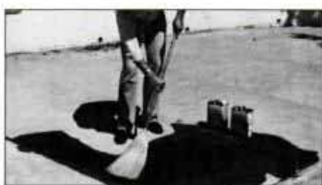
On stubborn stains, use a stiff broom to thoroughly mix the cleaner with the oil.
