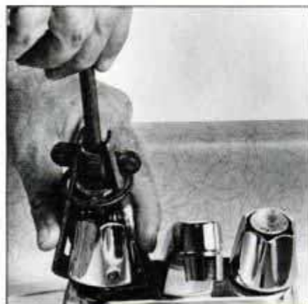
2 Remove faucet screw, then gently pry off handle with screwdriver. If stuck, use handle puller, as shown, to prevent damage.
