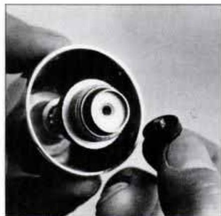
4 Remove worn washer from valve stem, then replace with new one. Tighten screw so washer just begins to compress.
