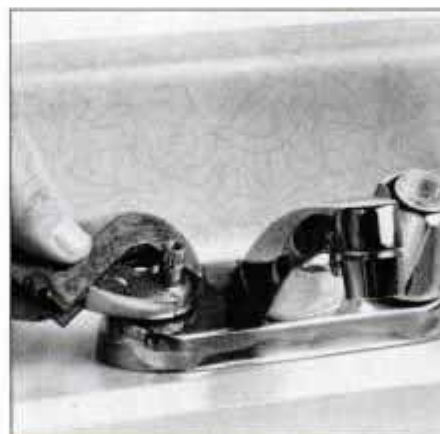
3 To remove valve stem, slide adjustable wrench over lock nut and turn counterclockwise. Valve stem should come out easily.
