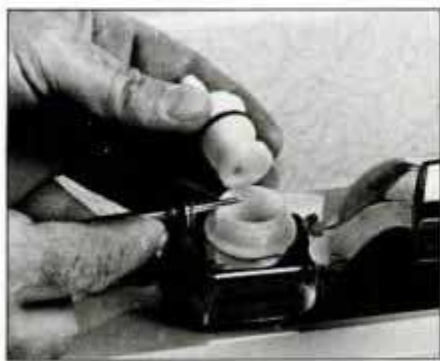
6 On washerless faucets, entire cartridge—including spring cup on bottom—must be replaced. Use awl to guide both.
