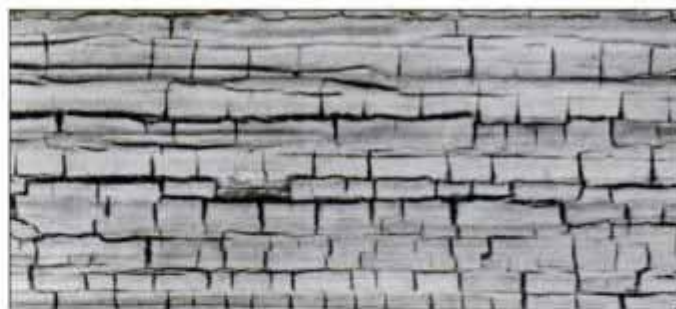
Alligatoring is caused by painting over a glossy finish.
