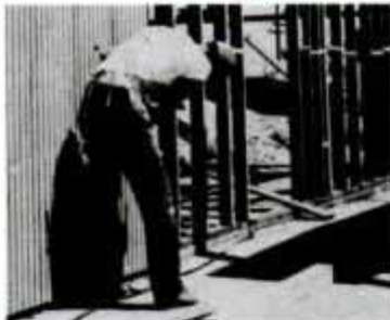
Exterior wall coverings can be installed with many different materials. Here's a texture 1-11 plywood siding panel applied directly to studs, thus eliminating the need for sheathing.
