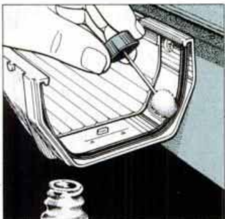
8 Apply silicone lubricant to gasket seals of slip-joints to promote smooth sliding action as the gutters expand and contract.
