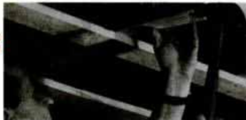
Covering an old floor with underlayment can be speeded up with a nailing machine. The book explains every step.
