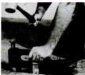
Metal diagonal bridging with nailing flanges can be used to keep floor joists well braced.
