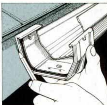
6 Here's a quick way to position slip-joint fittings: Align gutter end with insertion mark in fitting and pencil a line on fascia.
