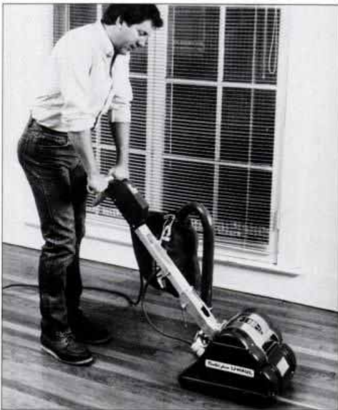
Use a rented drum sander and coarse sandpaper to begin resurfacing a wood floor. Make repeated passes in the grain's direction. Then sand with medium- and fine-grit abrasives.
