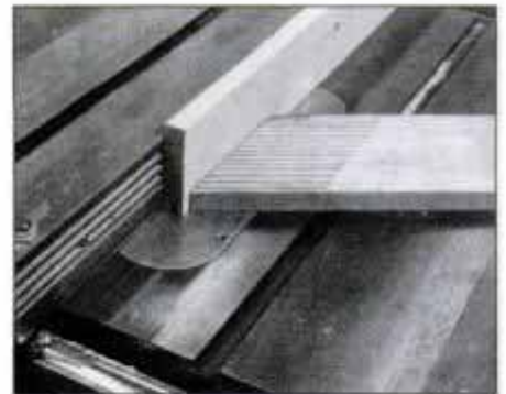
15 Cut \frac{1}{4} -in.-wide grooves in door rails and stiles with dado blade in table saw. Featherboard holds workpiece against saw fence.
