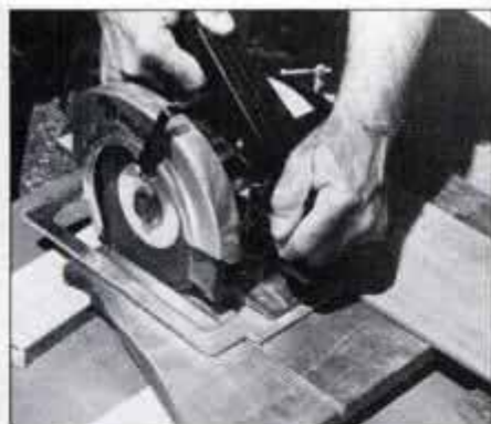
Use a silicone-carbide masonry blade to cut slate. Make the cut progressively; lower the abrasive blade slightly after each pass.
