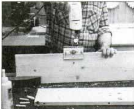
1 Bore \frac{3}{8} -in.-dia. dowel pin holes in board edges with the aid of a doweling jig. Masking tape gauge on bit acts as a depth gauge.
