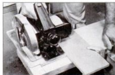
Then, use this dimension—in this case, 4\frac{3}{4} in.—to position the straightedge guide exactly parallel to the cutting line, as shown.
