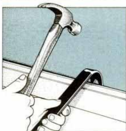
1 To remove baseboard, gently drive a pry bar between the trim and wall. Then pry board away at all nail locations.
