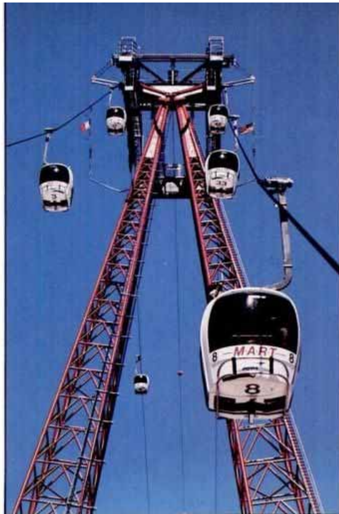
High-speed, lightweight lifts have broken more than speed records. In New Orleans, world's tallest gondola tower graced World's Fair.
