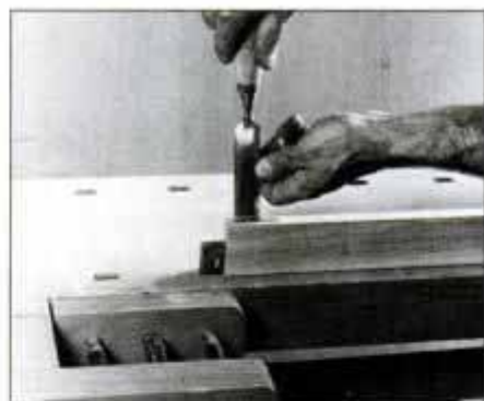
12 Use a sharp chisel to remove remaining waste from the mortises. Chisel the mortise walls smooth and square up the ends.
