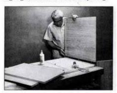
5 Begin assembly by gluing the end panel to the desk front. Dowel pins should penetrate the corner piece just 1/2 in.
