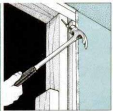
2 Assemble Jack post by nailing Jack stud to common stud at proper height. Toenall post to top and bottom wall plates.
