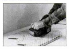
After all strips have been laminated to the underlayment, surface with a belt sander. Then trim the panel to its finished size.
