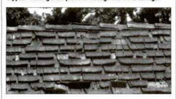
These wood shingles are showing signs of advanced weathering and should be replaced. Note how many of the shingles are split, cupped or have been blown off altogether. side of the roof. Condensing there, it can cause the rafters, and eventually even the roof deck, to decay. It also damages the roofing itself. In other cases, roofing materials simply suffer wear and tear from constant exposure to the elements.
