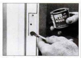
Stripped-out screw holes can be repaired with filler. First, enlarge the holes by boring them out, then fill them in and clean off excess.
