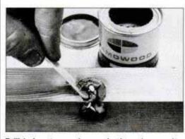
Drill holes at opposing angles in a deep cavity, then drive nails into them to provide "keys" for the filler. Fill the cavity and sand flush.
