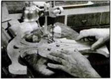
4 Scroll saw provides the easiest and most accurate means of making the cutouts in the chair back. Holes provide blade access.
