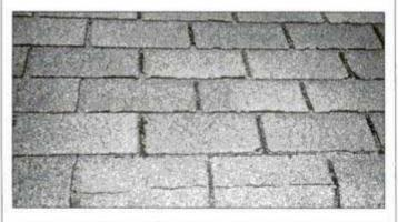
The asphalt shingle roof above needs replacement. Its mineral surface has worn off and the shingles are chipped, cracked and cupped—making them prone to leakage and wind damage.
