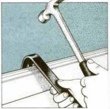
10 To gain access to wall cavity for running power cable, carefully pry baseboard from wall under new switch location.
