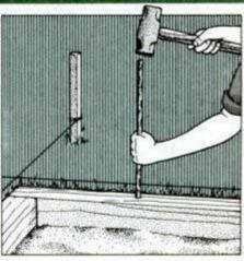
8 To stabilize beams, install lengths of reinforcing bar in each hole using a sledge hammer. Drive rebar flush to surface.
