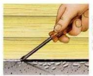
Over time, ordinary caulk cracks and falls apart. When that happens, it's time to remove the old caulk with a screw driver and replace it with a durable seal.
