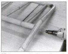
15 Clamp rear rail and crest pole together. Then join the end of the rail to the pole with glue and screws.
