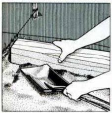
Adjust beams—relative to the string by adding or removing sand from underneath. Make sure beams do not rock.
