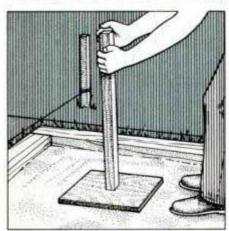
9 Install sand, rake smooth then spray with water. Compact sand with tamper made of ¾-in. plywood and 2x2 handle.
