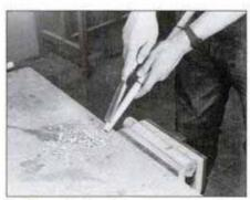
13 Cut spindles, then pare ends to ¼ in. dia. with sharp chisel. Test-fit in scrap rattan that has ¼-in. hole bored in middle.
