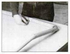
8 Use splice joint cut on first pole as template for marking joint cut on end of mating pole. Cut joint on second pole.
