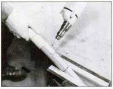
9 Join splice joint with glue and screws. Countersink heads so they can be covered with wood filler later.
