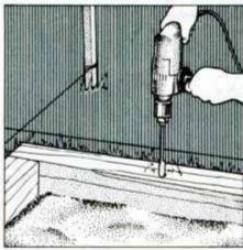
7 Once beams are laid, bore %-in.-dia. hole through beams at 2-ft. Intervals. Use spade bit in drill or auger in bit brace.
