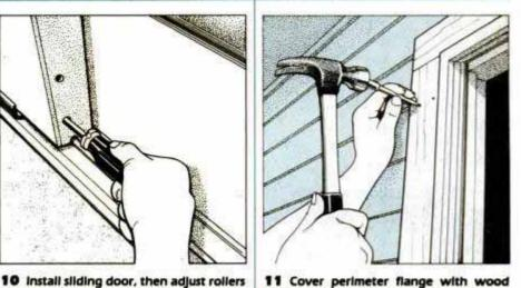
11 Cover perimeter flange with wood trim that fits between new door jambs and siding. Set and fill casing nailheads.
