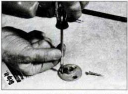
Once their holes have been bored, masonry screws are driven in the same manner as wood screws. They work with concrete, block or brick.
