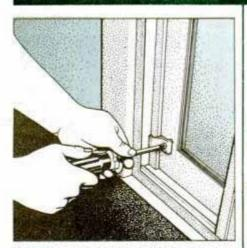
Begin by removing fixed door panel from old sliding unit. Usually, it's held by brackets screwed to the door and jamb.
