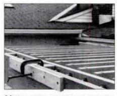
14 Use jig for boring pivot holes in middle beams. Bore first hole, insert dowel pin for alignment, bore other holes through jig.
