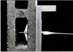
The toggle bolt threads through a nut in the wings, pulling them against the wall and tightening the wood against the masonry in a vise-like action.
