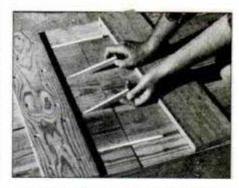
4 Join boards and cleats with screws to form storage compartment doors. Use ½-in.thick spacers to maintain alignment.
