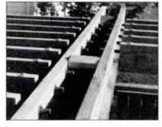
15 Install one set of louvers to stabilize structure, then install second set. Louvers must be pushed into middle beam holes first.
