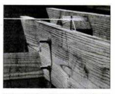
9 To make sure louvers align, attach string to end louver beams at point where louvers start. Mark middle beams under string.
