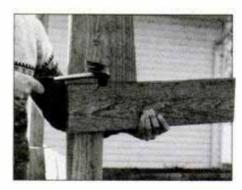
2 Cut seat supports to size, then tack-nall to post sides directly under back braces. Maintain 5° angle for best seating comfort.
