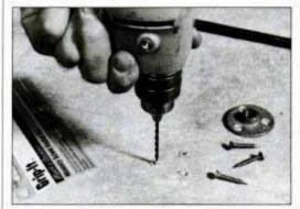
Self-tapping masonry screws are an alternative to cut nails and other wedge fasteners. Use a carbide bit, matched to the screws' size, to bore the hole.
