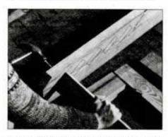
8 Cut screen uprights to size and shape, then set rail on edge and attach uprights at layout marks—using galvanized nails.
