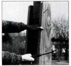
1 After posts are set in holes, plumb and brace them in place. Then begin seating benches by nailing back braces to post sides.
