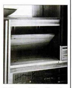
Leveling screws (4) in turntable panel are inset in rubber feet to dampen vibration.
