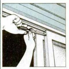
3 Next, loosen the alignment bracket on the top corner of the fixed door and pull bracket down. Door should now be free.
