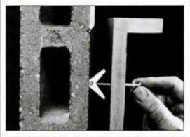
Toggle bolts excel for securing heavy loads to hollow concrete block walls. Their wings, pushed through the hole, expand on the other side.
