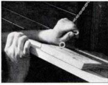
6 To support door in open position, attach screw eye to door cleat, then attach chain with spring snap hook to inside of post.
