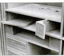
16 This view of center cabinet shows VCR compartment located beneath TV shelf. Note that TV shelf supports are removable to permit feeding the power cords.
