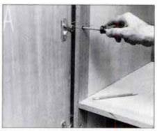
14 Screw the hinges to the mounting holes in the doors and then reattach the hinge to the sliding tracks. Adjust the hinges until the doors operate properly.
