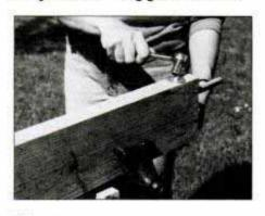
12 Secure tubing in ends of louver boards by installing bolt, washers and nut. Tighten bolt head with socket wrench.
