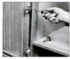
12 Attach the self-closing, fully adjustable door hinges to the sliding tracks. The screwdriver access holes permit easy installation, adjustment and disassembly.
