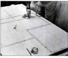
7 Remove cabinet and bore screw-shank clearance holes, spaced 8 in. apart, in center of the outlines. Use a drill-guide attachment to ensure perpendicular holes.
