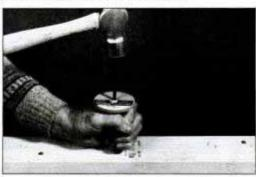
A heavy hammer is used to strike the drive rod. The pin, below it, is driven into the masonry. The top flange protects the user's hand.
