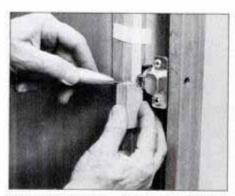
13 Here's how to transfer hinge centers to the doors. Use a notched block to mark hinge centers on wood strip. Then, use strip to mark hinge locations on doors.
