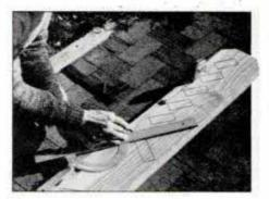
7 Cut privacy screen rails to size from 2 x 8 stock. Then lay out position of all screen slats using a protractor or framing square.
