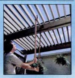
The overhead louvers are adjustable—using two easy-to-build tools—so you can regulate the sunlight that passes through.
