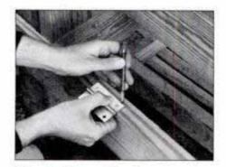
5 Locate hinge position for storage doors on rear support board. Then trace leaf outline and mortise board with sharp chisel.
