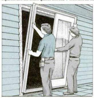
8 Lift new door frame into opening so sill comes down flat on caulk. Push top against wall. Don't slide bottom over caulk.
