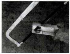
13 Cut aluminum louver channel to length. Then cut 2-in.-long notch in both ends to allow clearance for washers and cotter pins.
