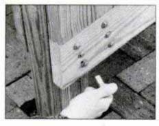
3 Prebore clearance holes, then attach seat supports using lagbolts and washers. Tighten until washers begin to depress wood.
