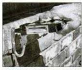
Fasteners anchor securely to brick. If pin doesn't drive flush, reposition, and shoot again.
