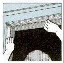
5 Once both doors and the door frame are removed from the opening, check corners of rough opening for square.
