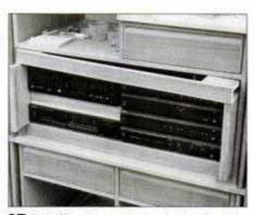
17 Install custom-cut panels to give the equipment a built-in look. Two components on left are separated by a platform to create two equal stacks of equipment.
