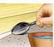
The trick to getting a smooth bead is to tool over the fresh sealant with an old spoon dipped in a soap solution. You'll have a professional-looking long-lasting seal to protect your house!
