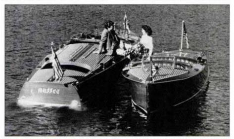
The Hackercrafts 30 (left) and 24 (right) in repose. Longitudinal seams are actually painted white. Metal hardware is cast from molds patterned after original equipment.
