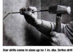
Star drills come in sizes up to 1 in. dia. Strike drill repeatedly with heavy hammer (2- or 2½-pound). Rotate bit 15° after each blow.
