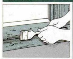
1 If old paint or other finish is loose on surface, first remove flaking areas with a scraper. Hold tool at low angle and pull.
