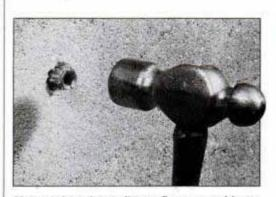
Most anchors have ribs or fins on outside to prevent turning in hole. Light hammer taps are required to bring anchor flush to surface.
