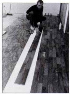
12 Longstrip Plank is a laminated product that comes in 5%-in.-wide x 8-ft., 3%-in.-long boards. Here, a full, uncut board is installed immediately after glue is applied.
