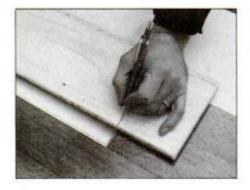
7 Here's a quick way to mark the last board in a row without measuring. Place one end against the wall separated by a ½-in. spacer. Then, mark the line of cut on the board.
