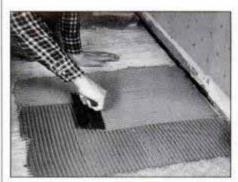
8 Spread mastic evenly over a small area using a %-in.-deep notched trowel. Leave chalk lines visible for tile alignment.
