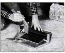
6 Wherever possible, cut tiles to size before spreading mastic. Cutter scores tile surface square, then snaps tile apart.
