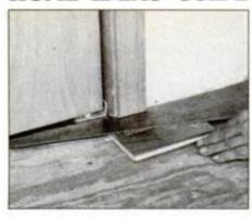
**3** Use a handsaw to cut existing door casings to accommodate the new floor. Use a section of the flooring and a piece of foam as a guide to determine new flooring height.
