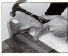
10 To close the end joint on the last board of each row, add a ½-in. spacer and then drive in a hardwood wedge. Leave spacers and wedges in place until the glue is dry.
