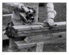
18 Cut angled mortise on top members of privacy screen by making saw kerfs. Clean out and flatten mortise with sharp chisel.
