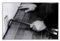
16 Rip the boards for the last course along the pencil lines using a portable circular saw or a sabre saw. Then, apply glue and use a crowbar to pry the edge joints closed.
