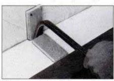
14 You can also install the second to the last course using a crowbar, as shown. Be sure to position the vertical wood block in front of a wall stud for maximum support.
