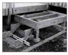
20 Frame step landing, then excavate for sleeper that supports stringers. Cut stringers to size, clamp in place, check for level.
