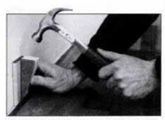
17 Once the last course is installed, add 1/2-In. spacer blocks and then drive in hardwood wedges, as shown, to close the edge Joint. Leave the wedges in until glue is dry.
