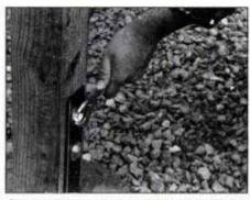
8 Cut wood posts to length and slide bottom and between column anchor flanges. Bolt in place using lagbolts and washers.
