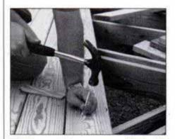
14 Once seat frames are complete, install decking across joists at 45° angle. To maintain alignment, use ¼-in. spacing blocks.
