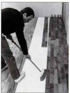
11 After installing each course, sweep the foam underlayment clean of all dust and dirt. Area under tongued edge must be clear of debris to ensure a tight-fitting joint.
