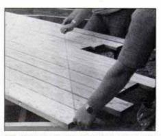
15 Allow decking boards to run over edge of deck. Then snap chalkline and cut ends in one pass to ensure precise alignment.
