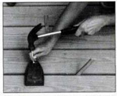
11 Nail decking in place using galvanized nails. To reduce wood splitting, blunt all nail points with hammer before driving.
