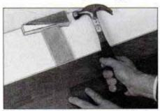
13 When installing the second to the last course, there won't be room to use a hammer and tapping block. Close the edge joint using two wedges and a wood block.
