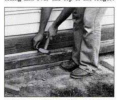
2 Transfer position of bolt holes to foundation using ledger as template. Slide punch or cold chisel into hole and strike with maul.
