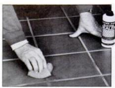
12 Replace baseboard and quarter round. After three days, seal grout with silicone sealer to protect it from dirt.
