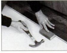
**6** Drive the joint closed using a hammer and a hardwood block. Tap the block in several places along the board's edge. Heavy pounding will damage the tongue.
