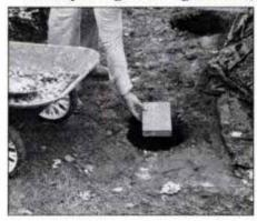
17 Excavate for privacy screen posts, then pour in 6 in. of gravel. Cover gravel with scrap 2x6 to support post. Backfill with soil.
