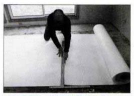
2 Cut the foam with a knife to fit from wall to wall. Here, an aluminum wallboard T-square is used to ensure straight, square cuts. Be certain to sweep the subfloor clean before laying the foam.
