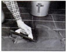
10 After mastic has set for 12 hours, spread grout using a rubber float. Force grout into grooves with float edge.
