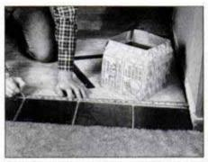
4 Lay out tiles, leaving appropriate grout spacing, to determine tile placement and the starting point for installation.
