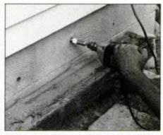
3 Bore matching bolt holes in foundation using masonry drill bit. Hole diameter and depth must match size of anchors.
