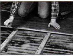
2 To keep the tile surface flush with the adjacent floors, cut at the joint line where the tiles will meet the floor. Remove the existing flooring in the area to be tiled.
