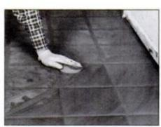
11 Wipe up excess grout, then strike joints with a smooth, round instrument. When dry, remove residue with burlap.
