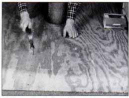
**3** Giue and nail down the exterior plywood subfloor to bring the finished tile surface to a fraction of an inch below the adjoining floor. Place the plywood's good face up.
