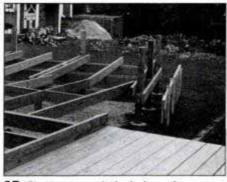
12 Construct angled decks using same methods as straight decks. Keep in mind that deck posts also support benches.
