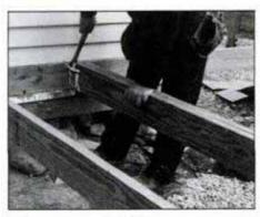
10 Attach decking joists to header joist with joist hangers. Note that header sits on top of flashing that covers top of ledger.
