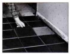
9 Begin first row along a central chalk line, then align adjacent tiles. Press so mastic squeezes out slightly at edges.
