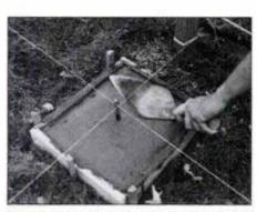
7 Flat-pad piers are laid out like round piers. But this time anchor bolts fall under string intersection, not column anchors.
