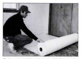
1 Cover the subfloor with 1/6-in.-thick foam underlayment. The foam provides a cushion for the floor, it silences squeaks and acts as a sound barrier. The foam is available in 5-ft.-wide rolls.
