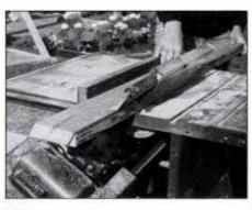
19 Bevel rail edges on privacy screen using table saw or portable circular saw. One side of top railing boards also needs bevel.
