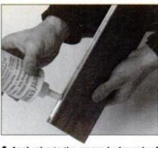
4 Apply glue to the grooved edge only of the first board. Be sure groove is clear of any debris to ensure a tight joint. Avoid overgluing to eliminate messy squeeze-out.
