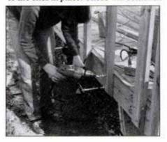
16 Bevel bottoms of railing posts, then damp in place and prebore clearance holes. Attach each with two lagscrews and washers.
