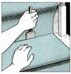
7 Work carpet tight around nosing, then into space between strips using a blunt cold chisel. Keep equal space between carpet edges and the wall and balusters.
