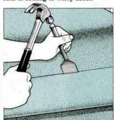
8 Drive the carpet into the crotch with the cold chisel to tighten carpet and secure it to tackless strips. Start from the center of the crotch and work toward each side.
