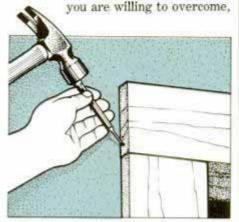
2 To save casing boards without damage, first see if the top board was toenailed into the sides. if so, drive these nails completely into the sides using a drift punch.
