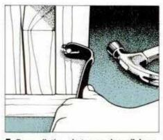
5 Once all the plaster or drywall is removed from the wall, pull out any visible nails using a nall puller. This simple tool is driven below the nailhead and pried back.
