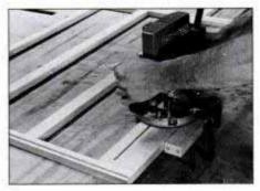
8 Cut spline grooves in back side of face frame using ¼-in.-dia. straight bit. Stop groove in bottom rail 2 in. from edge.
