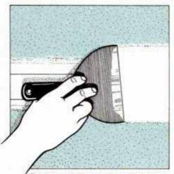
5 After tape is smooth, apply another layer of compound using 6-in. knife. Use just enough compound to cover tape.
