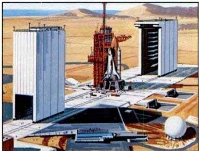
Space Shuttle will move from building to building on a flat car when the updated NASA Shuttle Launch Center is completed.
