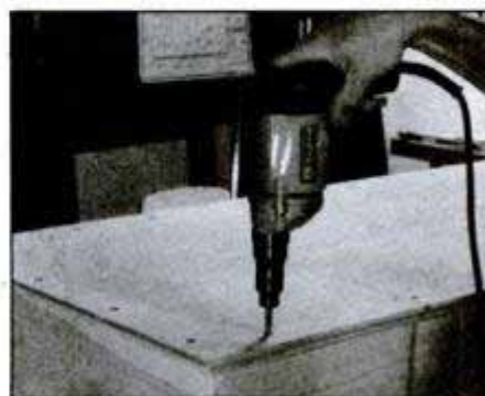
5 Once chest sides are assembled, center bottom over them and attach with screws. Be sure to bore and countersink pilot holes.
