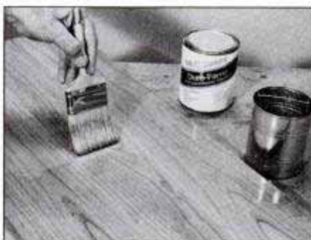
Tip-off the finish allowing only the bristles' tips to touch the surface. Strike wire on can is used to clean bristles of excess varnish.
