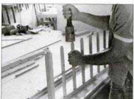
7 When grid assembly is dry, apply glue to grid tenons and frame mortises. Gently drive assembly in place with wood mallet.
