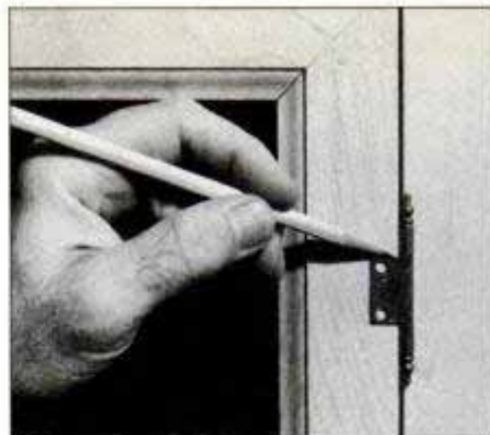
13 Attach doors with nonmortise hinges. For best alignment, hang outer leaf on case, then mark position of inner leaf on door.
