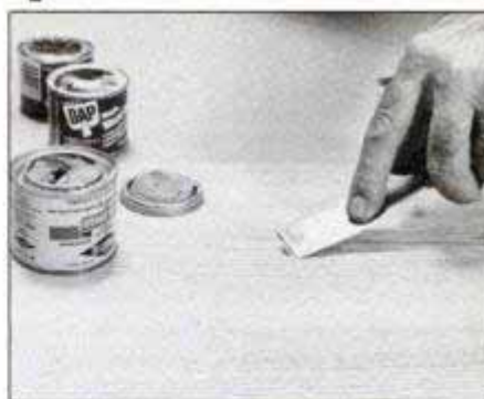
Fill small holes and gouges in the surface with wood putty (patching compound). Select a putty color that matches the wood.
