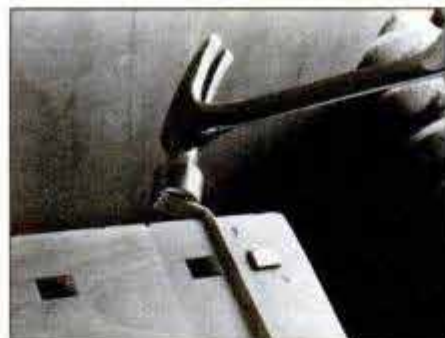
8 Clamp steel bar stock, for upper member of folding hardware assembly, into vise and bend over 1-in. section to a 90° angle.
