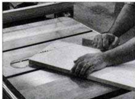
Mark the position of the slanted edges on bin sides, then make cuts with table saw miter gauge or radial-arm saw blade at 30°.
