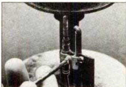
4 Remove the heater's thermocouple by loosening the screw on the retainer clip. Install the new thermocouple so that its heat sensor is in the path of the pilot flame.
