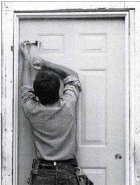
Unique Jamb-Jack fasteners (above, left) are used to attach the door frame to the rough opening. Screw the fasteners to the studs with a ratchet wrench (above, right).
