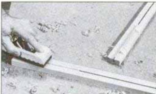
Glue and tape filler strip into lower portion of the dovetail grooves to plug them. Then, after glue dries, plane strips flush to surface.
