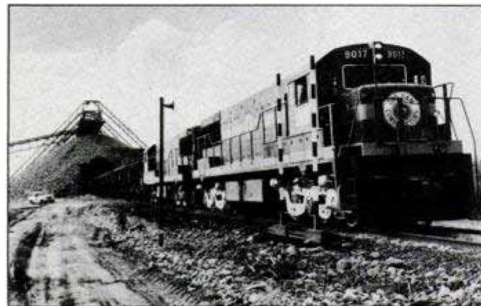
A special railroad line (left) was set up to move 120 carloads of dirt every hour. Excavation cars (right) carried mounds of dirt.
