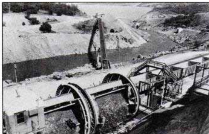
A special railroad line (left) was set up to move 120 carloads of dirt every hour. Excavation cars (right) carried mounds of dirt.
