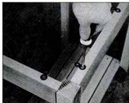
Attach tabletop fasteners to aprons using \frac{3}{8} -in. No. 8 fh screws. Note how fastener mortises intersect inside edges of aprons.
