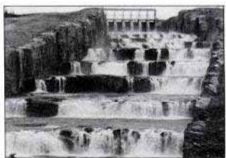
Water spills over a series of dikes at Hydro Quebec. The project uses 198 control dikes.
