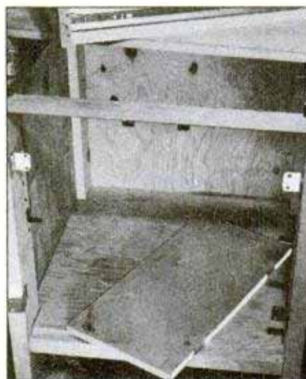
Flush doors butt against edge of cabinet bottom, and are held with catches at top. Plug-in clips support adjustable shelf.
