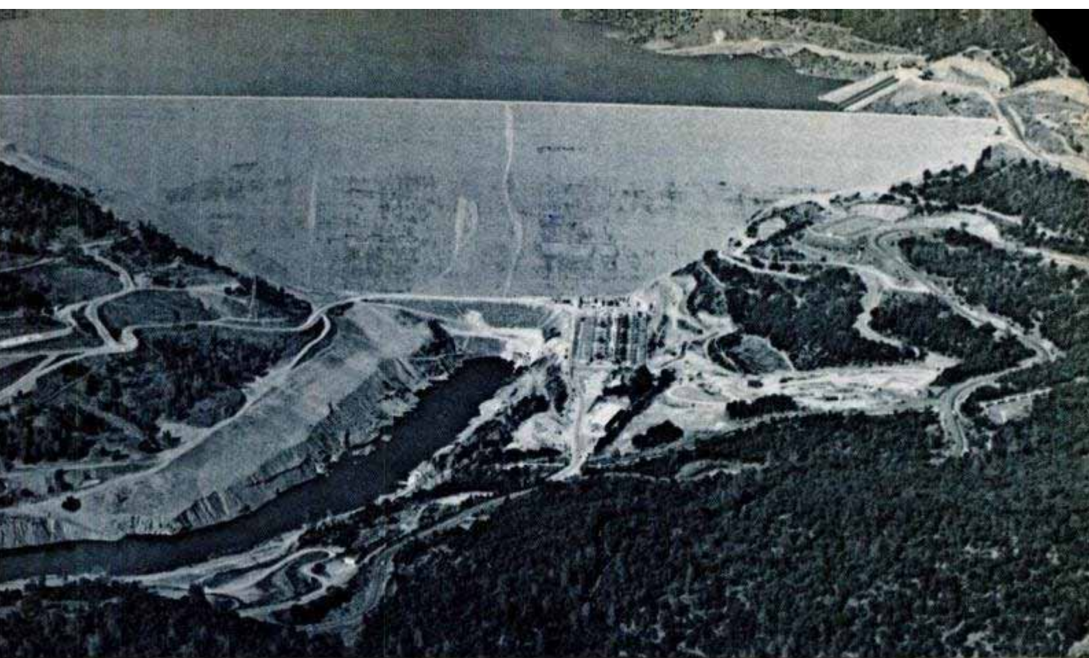
Oroville Dam is seen at end of construction in 1967 (above). Dam is 770 feet high. Spillways (far left) have a series of gates to control water flow precisely. Work crews carved out a 69-foot by 500-foot cavern (left) 600 feet below ground to house a generating plant.
