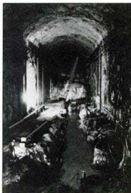
Oroville Dam is seen at end of construction in 1967 (above). Dam is 770 feet high. Spillways (far left) have a series of gates to control water flow precisely. Work crews carved out a 69-foot by 500-foot cavern (left) 600 feet below ground to house a generating plant.
