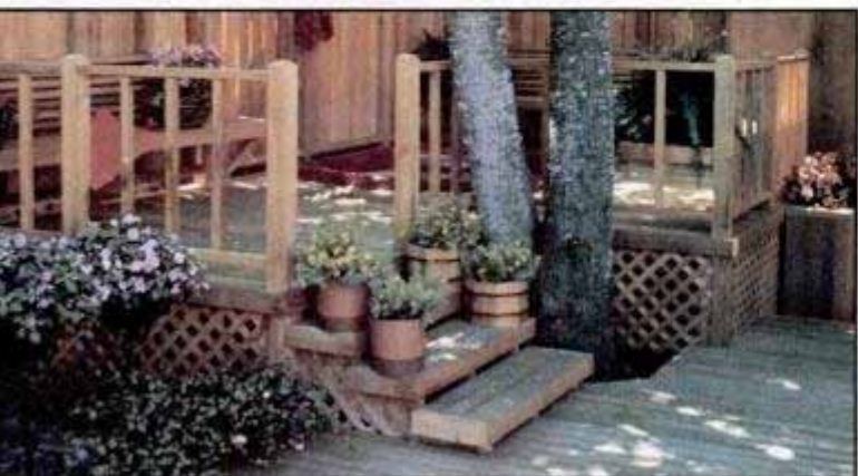
3 Three steps form the transition between the two decks. The lattice skirt on the upper deck hides the framing underneath.
