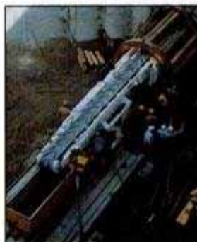
Cross section above shows how ring of concrete "logs" encases three-level tunnel. At left, a 55-ton boring machine digs perimeter tunnels.
