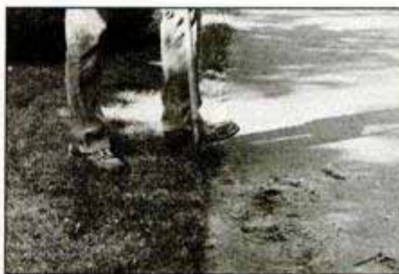
Sealing a blacktop driveway regularly protects it from weather and wear. Holes and cracks should be patched and allowed to cure before the sealer is applied.
