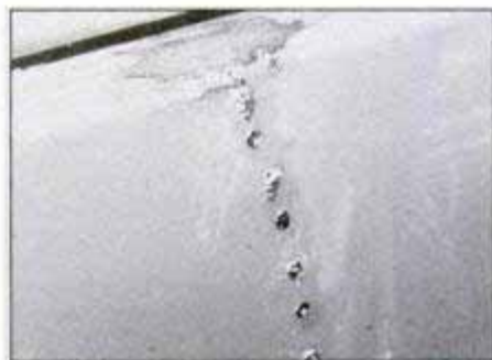
Properly done, solder will flow around the tip of the gun and form a glob on both sides of the hole. Sand and repaint.
