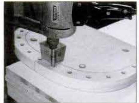
Cut angled guide block for each seat hole. Then, clamp each in place next to hole. Bore hole using corner edge of block as guide.
