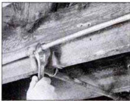
Thread the copper pipe and adapter assembly into the iron pipe supply line and tighten it securely with an adjustable wrench.
