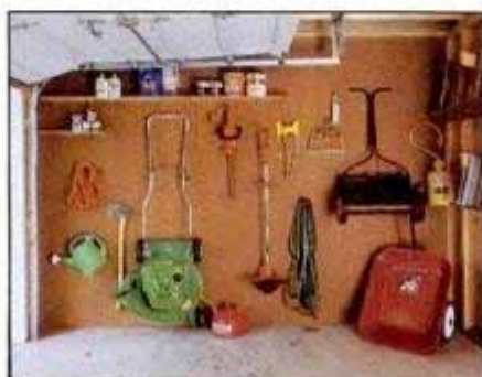
Interior of one side wall is covered with perforated hardboard to gain maximum storage room. With heavy-duty fasteners, even a lawn mower can be stored flat.
