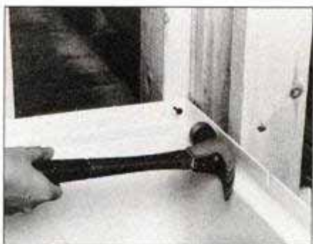
Prebore clearance holes in base flange, then nail flange to studs using 1½-in. roofing nails. Do not strike base with hammer.
