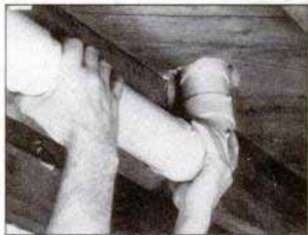
Test-fit preassembled section between the flange and the waste line. Then clean and cement both end joints at the same time.
