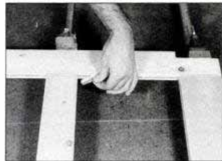
Glue small hardboard block into front and rear corner post grooves—just below middle side rail—to provide additional support.
