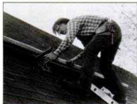
Position roof brackets below area to be cut using dowel as reference. Attach by lifting up shingle tabs and nailing directly to roof. Then, lay sturdy plank across brackets.
