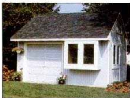
The front of this shed features a bump-out bay window made of two casement units and a 7-ft.-wide overhead garage door to provide easy access for garden tractors.
