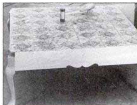
Set tiles in adhesive beginning at one corner, and following edge marks. Tap with mallet to achieve a uniformly flat surface.
