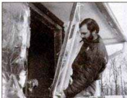
Pry out the window top first. Grip window frame and pull the unit from house. Keep window closed to make the unit more rigid.
