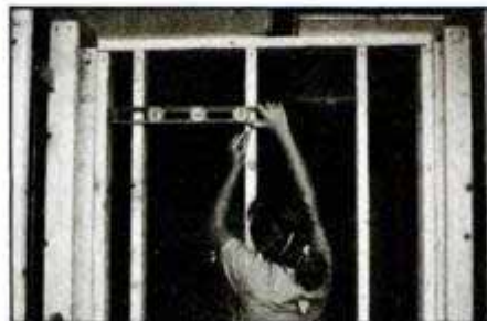
Draw level line across studs to position solid blocking behind flanges at top of walls.
