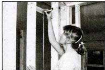
Install plumbing adapter in wall for shower head nipple so nipple falls above side wall.
