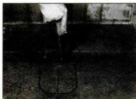
Cut the waste flange hole using a key hole, sabre or reciprocating saw. Make sure there are no wires or water pipes below the cut.
