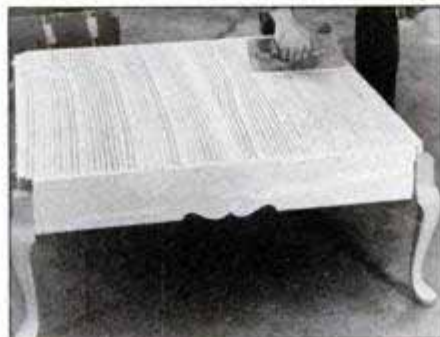
Lay tiles on top with even spacing, mark along outer edges and remove. Then apply adhesive evenly with a V-notched trowel.
