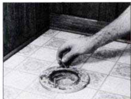
Slide the hold-down bolts into the flange slots so both are parallel to the room wall. The slots have room for precise adjustment.
