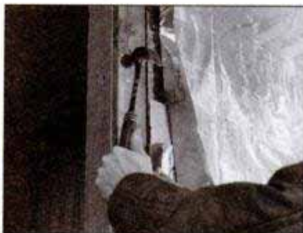
Nail stock to the house to bring the sheathing flush with the opening. Use material that is the same thickness as the sheathing.
