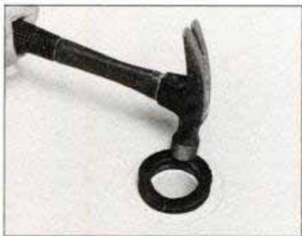
Lower base into former position and center hole around pipe. Press seal into hole and around pipe. Tap in place with hammer.
