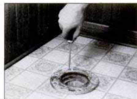
Align the flange on your new flooring so the hold-down bolt slots face to the sides. Attach with screws driven into the floor.
