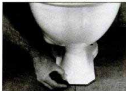
Make sure the bowl is square to the wall and centered over the floor line. Outline the entire base perimeter on the floor.
