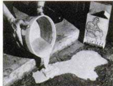
Anchoring and patching cement can be mixed for pouring, as shown, or to a pliable consistency for knife or trowel application.
