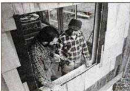
Truini and dad do a window installation.
