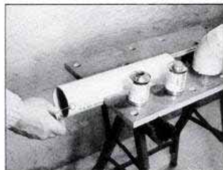
Next, apply plastic welding cement to the mating surfaces of the pipe and fitting using the applicator that comes with the can.
