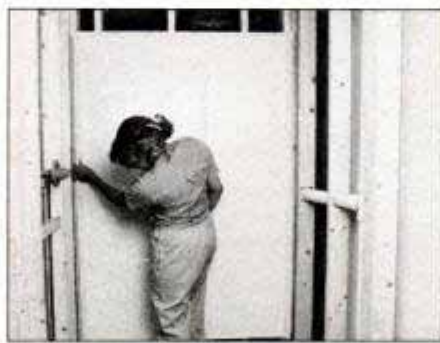
Lift rear wall into position then carefully lower into base alignment channel. Push from top so wall is seated uniformly.
