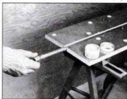
Also apply soldering flux to the inside of each fitting—in this case a male pipe thread adapter—and slide it over the tubing end.
