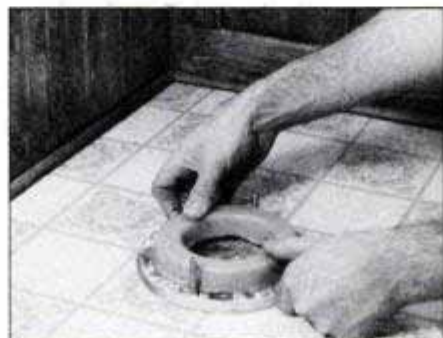
Press a new wax seal, smooth side up, onto the flange. It should fit just between the bolts and be centered over the waste hole.
