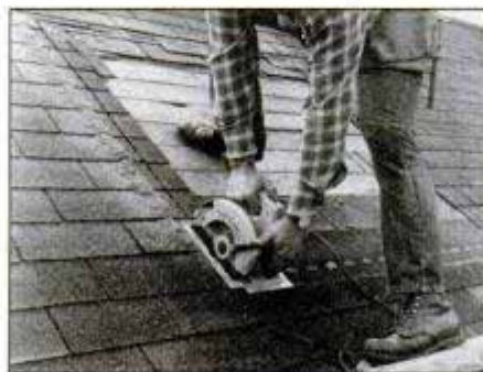
Remove shingles from interior of rectangle, then cut through roof sheathing using carbide blade in circular saw. Set blade depth so cut is just below bottom of sheathing.
