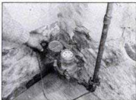
Begin by turning off the house water supply at the water meter. A valve should be on either the main side (above) or house side.
