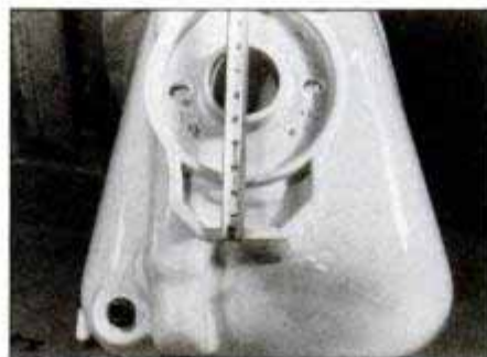
Stand the bowl on end and measure the distance from the back of the bowl's base to the edge of its outlet horn (center hole).
