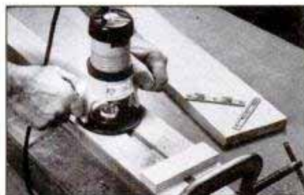
Clamp the platform jig to the bed post for routing the plate mortise. Be certain that the plate mounts flush to the post surface.
