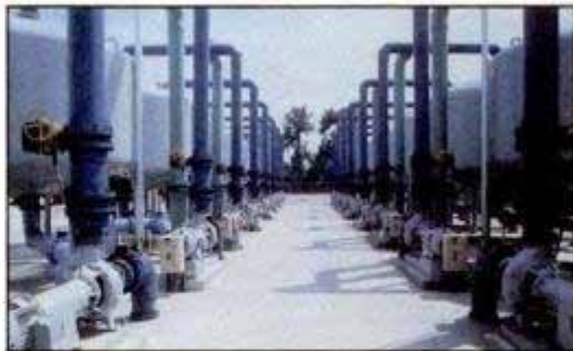
Chiller tower (above left) circulates one-third of pool water to cool it to 55° F. Sand filters (right) remove hundreds of pounds of waste.
