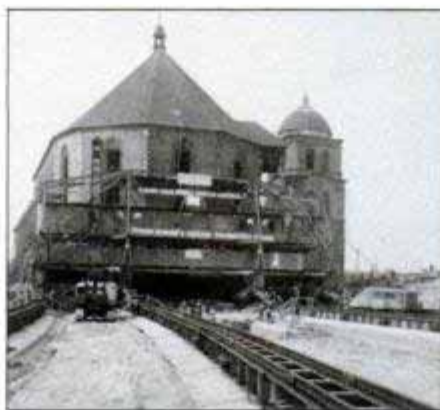
Moving a church: Better founded upon a rock than on a prime deposit of coal.
