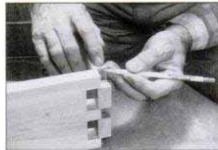
Test-fit joint frequently to check progress. Mark any high spots with soft pencil, then carefully shave to fit using sharp chisel.
