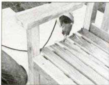
Join seat slats to side supports and front rail with glue and screws. Bore pilot holes and countersink head \frac{3}{8} in. deep. Use \frac{3}{4} -in. spacers between slats for positioning.
