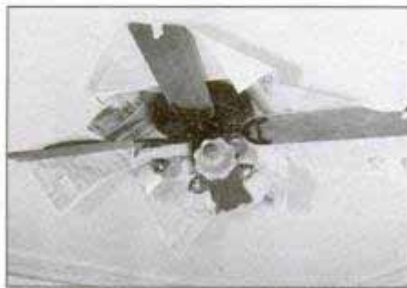
If you can't remove a fixture such as a ceiling fan or light, cover it with newspaper or plastic to avoid paint splatters.
