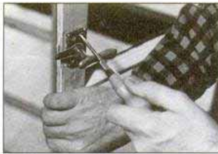
Remove hardware rather than taping it and trying to paint cautiously around it. It's faster and you get a smoother paint job.
