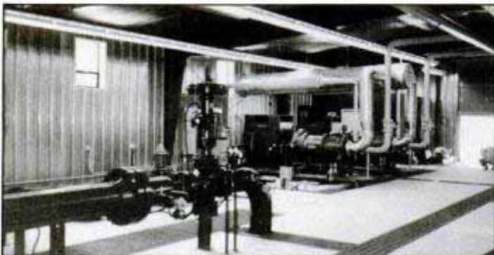
Single water pipe and set of cooled compressed-air pipes are housed in artificial snow shed (left). Computerized snow gun (above) sprays finished product. Water for the process is chilled (right) before entering system.
