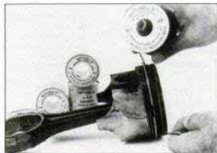
Abrasive cords scour hard-to-reach grooves.
