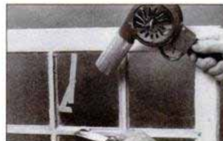
To remove hardened glazing putty, first soften with heat then peel off with putty knife. This prevents damage to wood caused by chipping out with a chisel.
