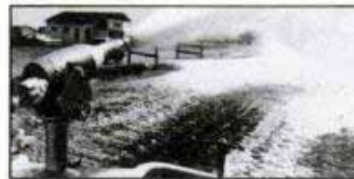
Single water pipe and set of cooled compressed-air pipes are housed in artificial snow shed (left). Computerized snow gun (above) sprays finished product. Water for the process is chilled (right) before entering system.
