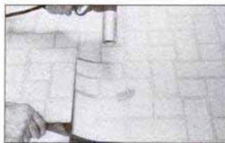
A damaged vinyl floor tile can be removed without harming surrounding tiles. Direct hot air at one corner until adhesive softens. Work putty knife under edge.
