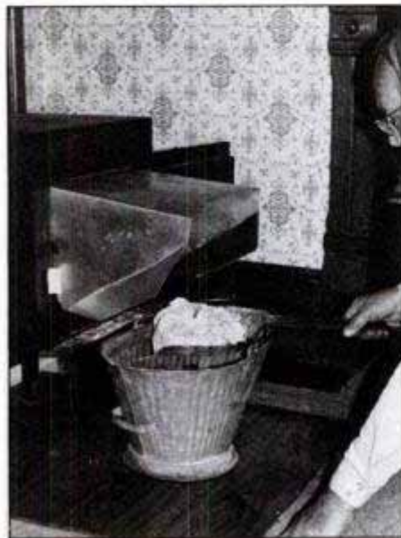
A sheet-metal hood over the stove opening channels ash dust to the ash receptacle.
