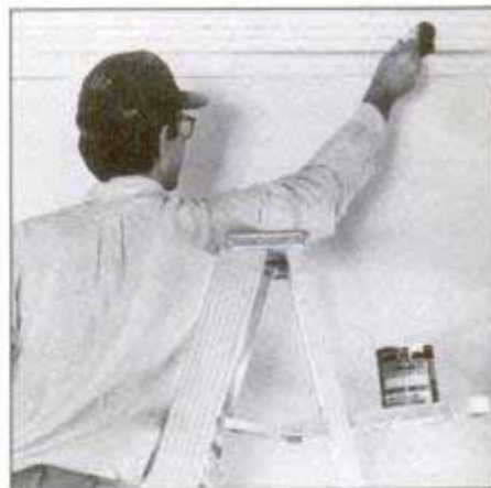
Check ceilings for water stains. Seal the stains with shellac or pigmented shellac so they don't bleed through the paint.
