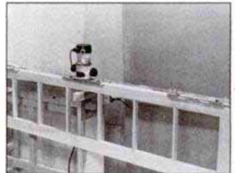
Door butt hinges must be mortised into stile edges. Router template above gives quick, professional results, but hand mortising with a sharp chisel will work as well.
