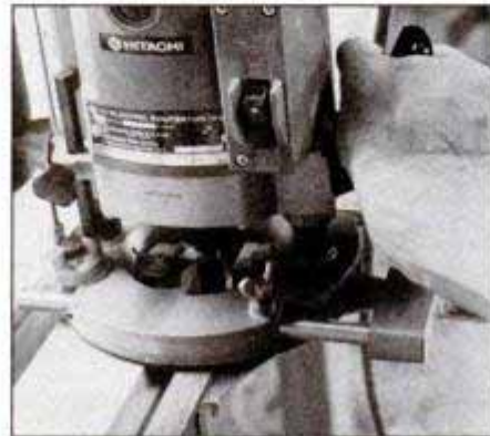
Rout matching rabbets on opposite sides of door stiles using \frac{3}{4} -in.-dia. straight cutter.
