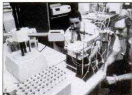
Purdue University robot is programmed to perform multistep chemistry experiments.
