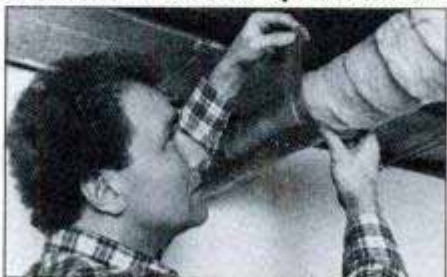
Wrapping insulation around water pipes in an unheated basement or crawl space keeps them from freezing during cold months.
