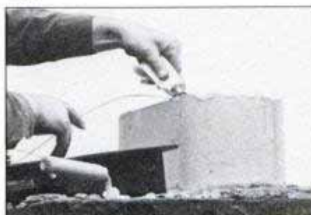
Apply two beads of the silicone rubber adhesive included in the kit to the top edge of the flue tile. The adhesive cures in 24 hours to bond the damper in place.
