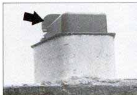
Press the damper in place. Make certain that it is working smoothly by opening and closing it several times. The spring-loaded lid (arrow) should remain open.
