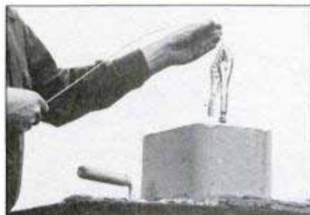
Use a Vise-Grip pliers to weight the cable that moves the damper. Lower the cable from the chimney to the firebox. A helper below can alert you when cable is visible.
