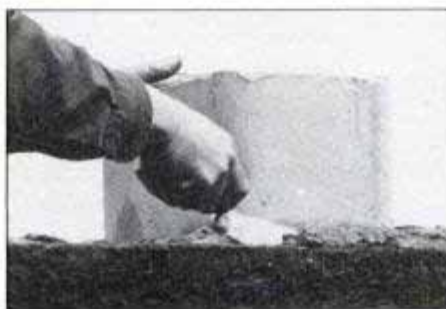
After removing hardware cloth or chimney cap, install flue tile. Use ready-mix concrete or mix mortar to pudding consistency and apply with a trowel around the tile.
