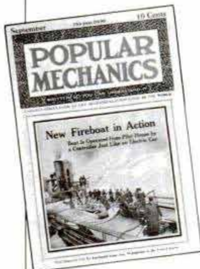
Fireboats run on electricity.
