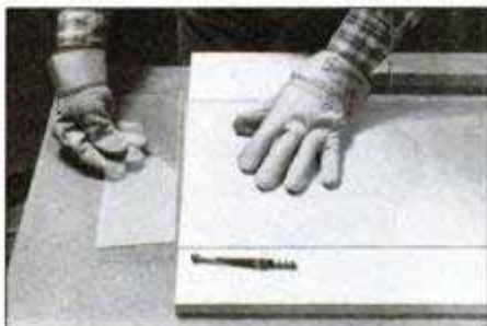
Move the score line over the edge of the cutting surface and snap the glass with a quick downward motion. Wear gloves when handling the glass to prevent cuts.
