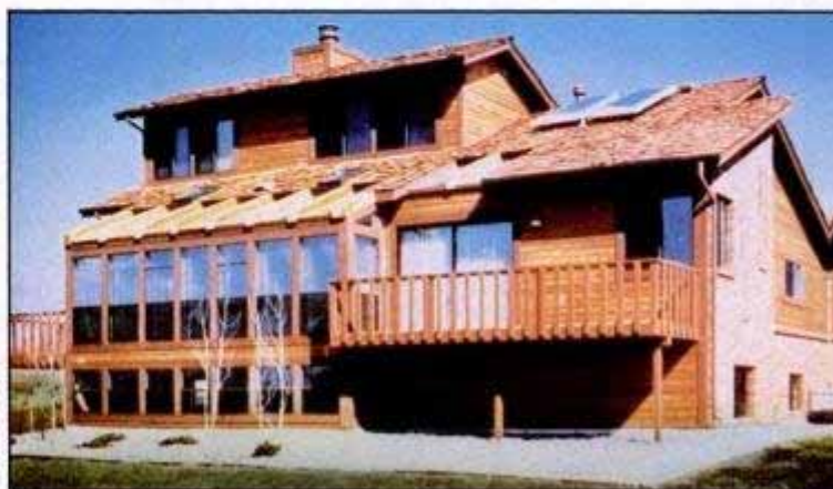
Denver-area house studied by the Solar Energy Research Institute could draw most of its heat from a south-facing sunroom. But tests show heat circulated only when sunroom doors were open.
