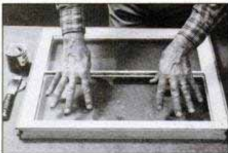
Apply a \frac{1}{8} -in. bead of compound across all rabbets to form a tight interior seal and to act as a cushion for the glass. Lay the glass in place; press evenly into compound.
