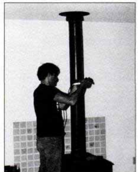
18. Slide the stove into place, install the stovepipe connector assembly and secure the pipe joints with sheet-metal screws.
