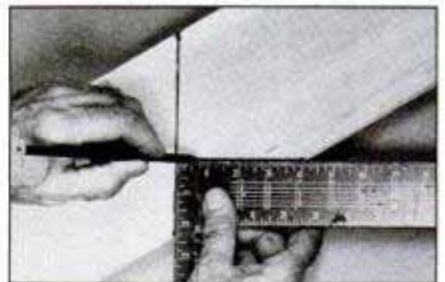
6 Hold square body perpendicular to lower plumb line and move up until 4-in. mark intersects bottom edge of rafter.
