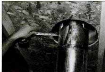
13. Besides checking for clearance, make sure no chimney section joints will be located inside a penetrated ceiling or wall.
