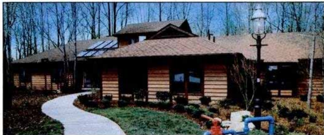
American Gas Assn. house in Cleveland has a two-story core and two experimental wings. It takes advantage of basic solar design, facing a true solar south. AGA began using the house this summer to test heating, cooling and cooking appliances.
