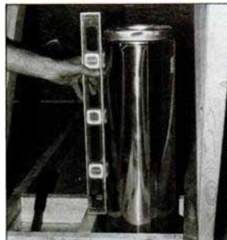
7 Place the first chimney section into the support base. Check the chimney for plumb. Add sections to approach roof.
