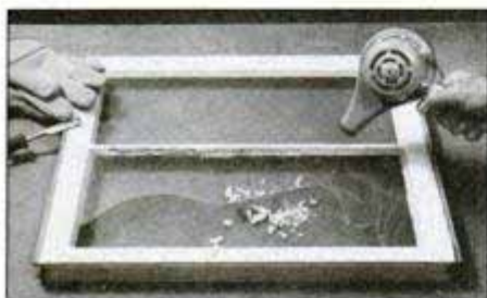
If the compound is too hard to chip away easily, use a hair dryer or flameless heat gun to soften it first. Be careful not to char the sash when using the heat gun.
