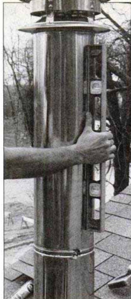
Careful installation of a metal factory-built chimney involves much less labor than the construction of a masonry unit.
