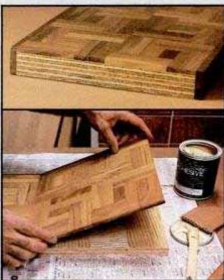
7. Parquet flooring —Glue hardwood parquet flooring to a plywood base. After assembly, add trim around the butcher block to conceal the plywood edge (top).
