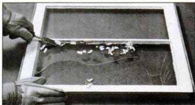
Remove loose glass pieces; then use an old but sharp chisel to chip off the hardened glazing compound. Do not gouge the frame.
