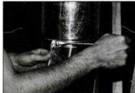
14. If locking bands are required according to the assembly instructions of the chimney manufacturer, install them.
