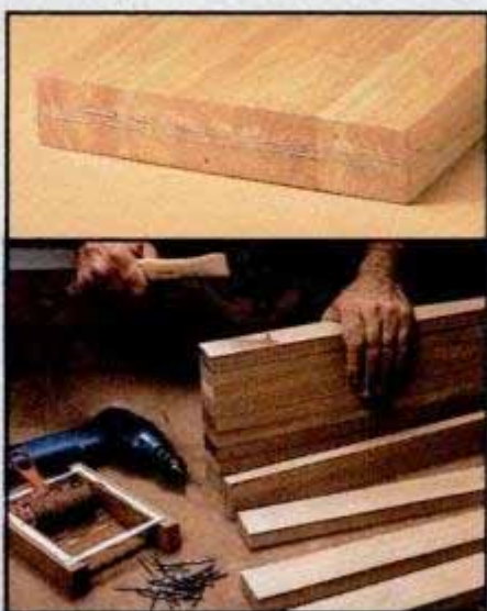
6. Direct-nailing —Here's a quick and easy way to make a strong joint. Simply glue and nail one board to the next until the desired width butcher block top is formed.
