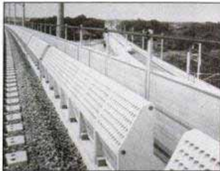
Calmzone barriers are being tested at commuter railroad tracks near Los Angeles (left). The structures (right) stand less than four feet high. Made of synthetic resin, the tapered and ribbed barriers are designed to damp and reflect sound waves.
