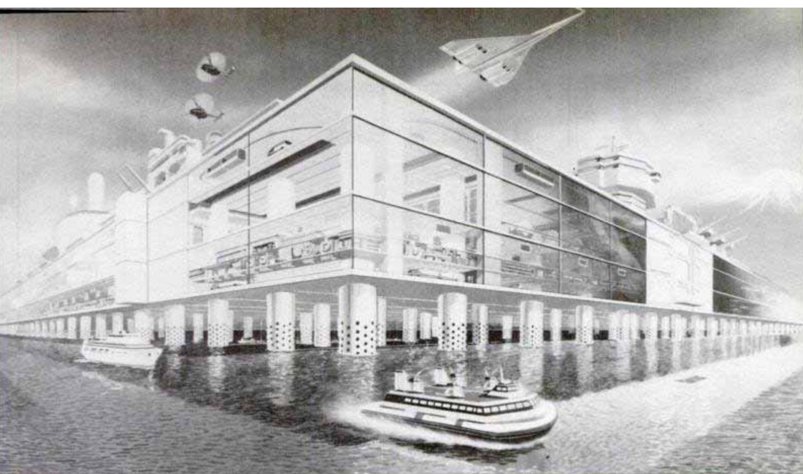
Mitsui Engineering concept of Tokyo Harbor Airport Island is based partly on early work of Buckminster Fuller. The island will stand on prestressed concrete pillars sitting on concrete pads that act as "shock absorbers" to keep the structure standing in an earthquake. Because the island will be raised above sea level, boats will be able to pass underneath.
