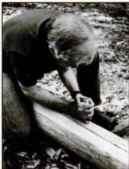
After rough bark is removed, the white bark that's left is scribed with a knife.
