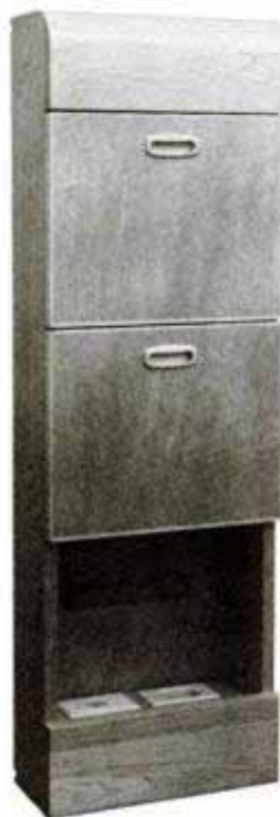
Finished cabinet is shown ready for installation. Note the clock outlet with recessed receptacle placed next to the phone jack.
