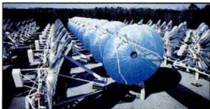
On a sunny day, the parabolic solar collectors generate 400 kw.
