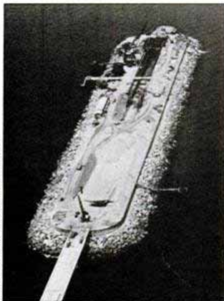
Artificial Island of Chesapeake Bridge-Tunnel is seen during construction.
