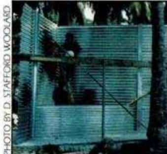
Tuvalu house uses ribbed aluminum to replace scarce thatch.
