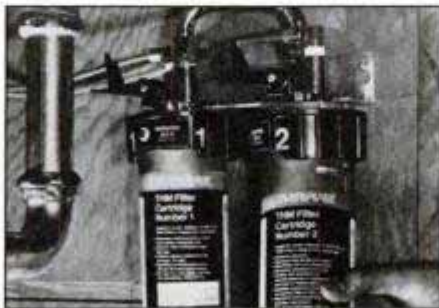
10 Shut off water filters by moving black handle counterclockwise as far as possible. Install filter cartridges (No. 1 on left). Turn tap valve handle clockwise to pierce water line; reverse for water flow.
