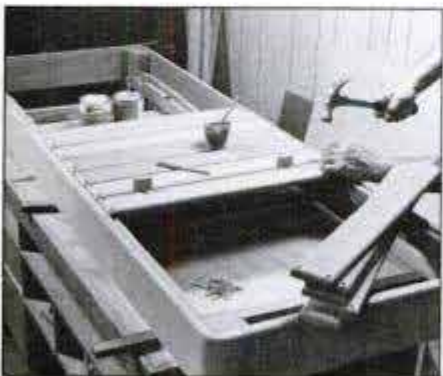
Glue and nail slats into place using drift punch to set heads and two 1/4-in. blocks to maintain even spacing. Nails in block centers keep blocks from falling.
