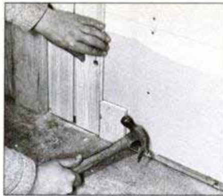
Drive next board into place so groove fits over first board's tongue. Use scrap block of wainscoting to prevent damaging edge. Nail second board through tongue only.
