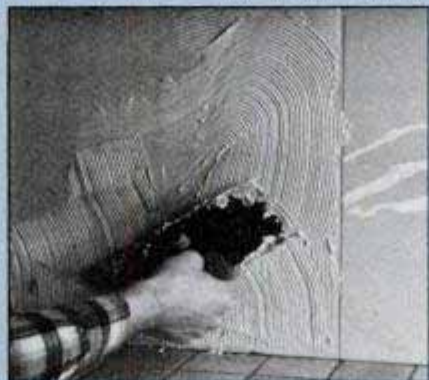
Use the smooth edge of the trowel to spread adhesive so that the vertical line remains visible. Then hold the trowel at a 45° angle and comb the adhesive.
