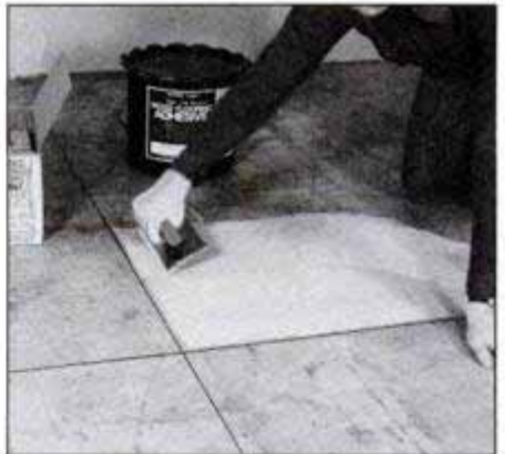
Apply parquet tile adhesive along the intersection of the chalklines. Spread only enough for about 10 minutes of work, to allow time for properly aligning tiles.
