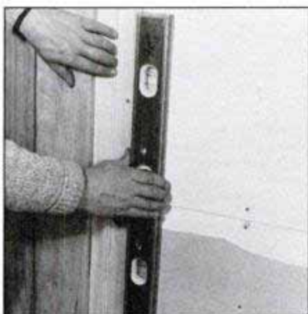
Start installing boards at room corner or door casing as shown here. For pro results, use level to plumb first board in place. Mark plumb position for reference.
