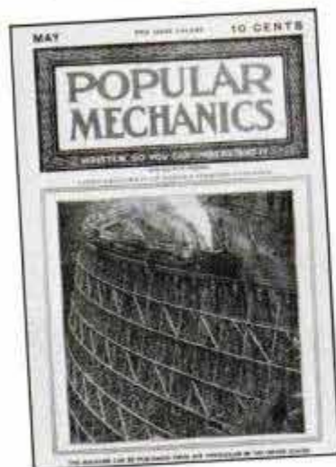
A new trestle made of timber.
