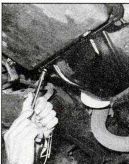
5 Drop the dust cover from the bottom of the transmission bellhousing section to reach the torque converter bolts.
