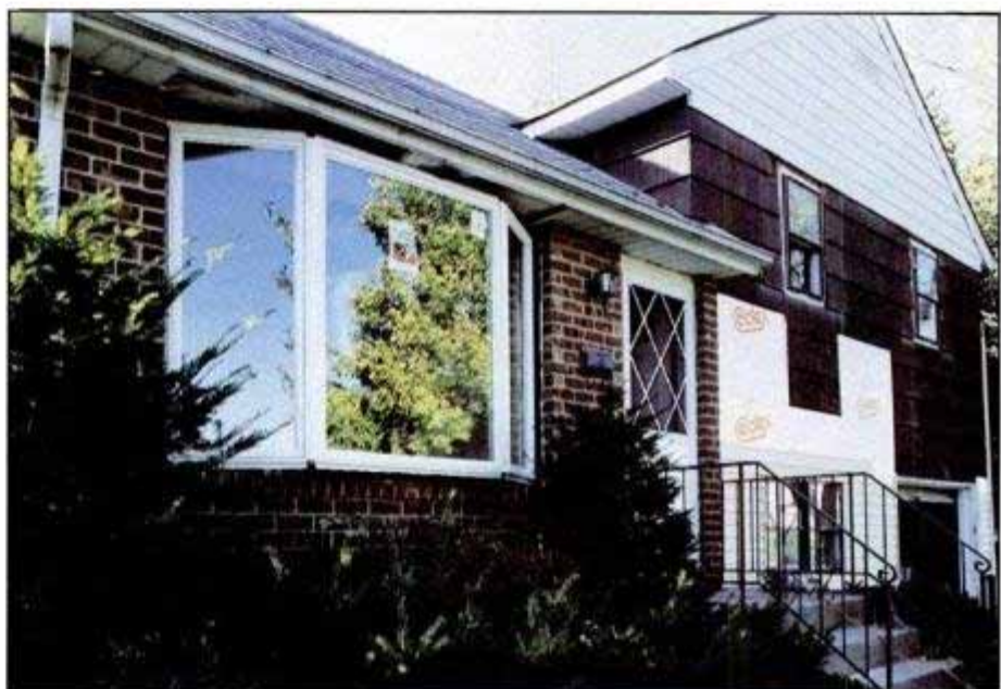
New bay and double-hung windows are in place. Rigid insulation and siding have been installed on the first floor. Scaffolding will be needed to work on the second floor.
