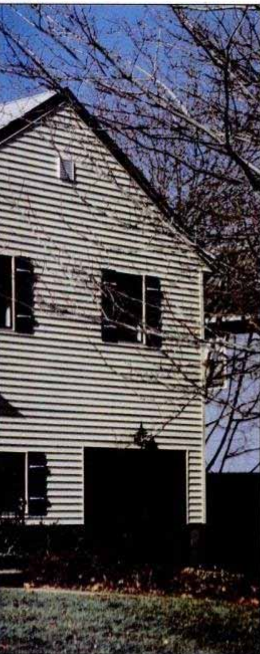
New bay and double-hung windows are in place. Rigid insulation and siding have been installed on the first floor. Scaffolding will be needed to work on the second floor.
