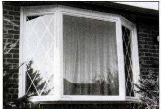
We ripped 2x4s to size for side fillers and nailed them in place. Then we nailed furnished angled side flanges. We bent aluminum to cover the wood trim and secured it with finish nails.
