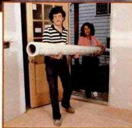
The kitchen flooring (top) is sheet vinyl that lies flat without adhesive. You should bring the flooring indoors (above) at least 48 hours before you plan to install it.
