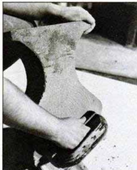
Rub the surfaces with a concrete finishing stone or sharpening stone to work up a paste that fills small voids. Brush remaining paste lightly for a smooth finish.
