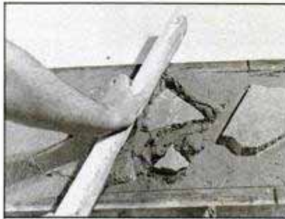
Dig out holes for the inlay pieces, then place pieces in holes and level them with a straightedge. Fill in around the pieces as you work across the top.
