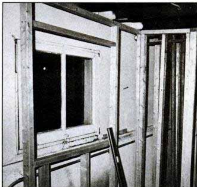
While framing out the basement walls, build a rough opening around the window that is at least 2 in. larger on all sides.
