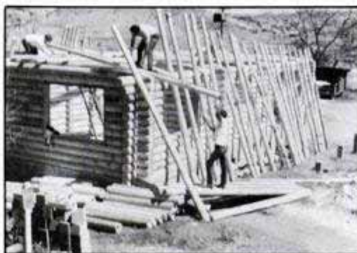
Several men following the stacking plan of a pre-cut log house can assemble the unit in a few days.
