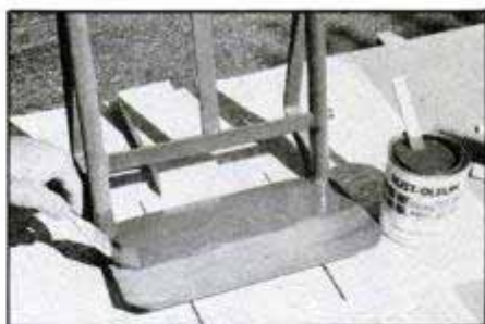
On extremely rusty projects, like the hand truck above, complete rust removal is too difficult. Instead, brush off the loose rust with a wire brush, then apply rusty-metal primer. Its fish-oil base penetrates through rust and drives out all of the air and moisture.
