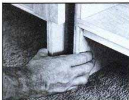
Space between bottom shelf (B on drawing) and floor is usable if a hatch is built in.
