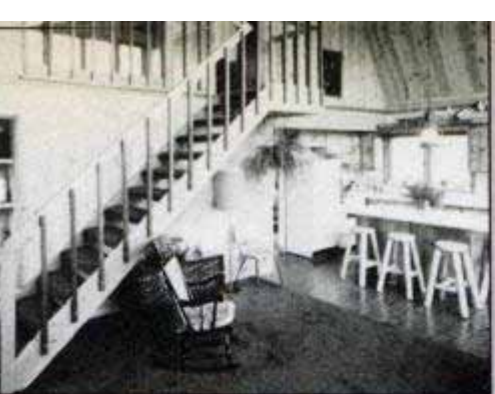
The interior parts of this house, such as the stringers, treads and banister of the staircase, are delivered cut and ready for assembly. Later, stairs will be carpeted. This precut house was made by Lindal Cedar Homes, which is in Seattle.
