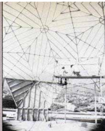
The basis of this dome's framework is the triangle, which is repeated six times around each hexagon (left). An example of dome hardware (above) is Timberline's steel straps. They are welded to a center ring and sandwich each wooden member.
