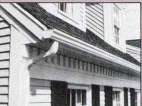
Careful eave and rake detailing, which includes precut dentils, is designed into this panelized house to give it a custom look. The house is by National Homes.
