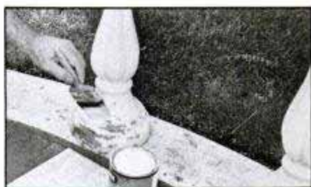
Before painting masonry, remove all peeled paint, grime and mildew. Use a stiff brush and a solution of 1 cup bleach, 1/2 cup detergent, and 1 gal. water. Allow to dry, then spot-prime the exposed masonry with an alkali-resistant acrylic primer.
