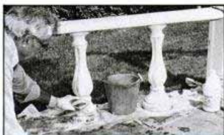
Before painting masonry, remove all peeled paint, grime and mildew. Use a stiff brush and a solution of 1 cup bleach, 1/2 cup detergent, and 1 gal. water. Allow to dry, then spot-prime the exposed masonry with an alkali-resistant acrylic primer.
