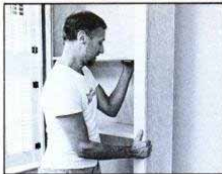
First box of five is placed in position in left-hand corner of room; others follow in line.
