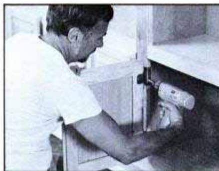
Attach the cabinet doors with self-closing hinges mounted on the cabinet stile edges.
