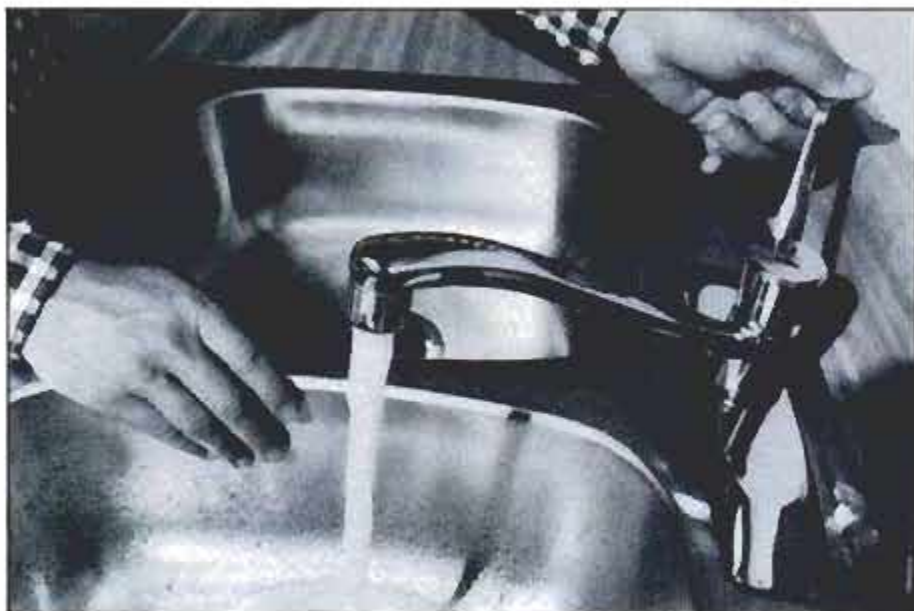
The fast shutoff of a modern single-lever faucet can lead to water hammer. When you install a new faucet, you should also consider adding air chambers to guard against hammer.
