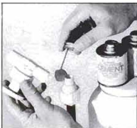
Solvent-weld line valves with waste outlets as shutoffs. Be sure the flow arrows point upward. The undersink parts must provide transition to the plastic, incorporate air chambers, furnish shutoffs and reach up to the faucet to connect it.
