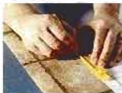
2 Transfer the pattern to your new floor.
