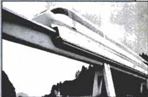
Transrapid guideway is elevated 16 to 20 feet above ground on concrete pylons.
