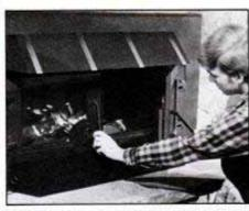
A fireplace insert turned the fireplace in the family room from an energy waster into an effective heat source. It can contribute up to 50,000 B.T.U.s of heat an hour.
