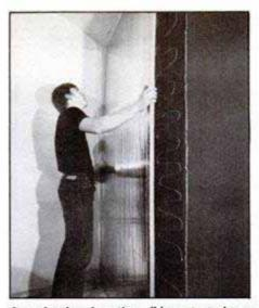
An uninsulated north wall is protected easily with rigid insulation installed over the drywall. Gypsum wallboard at least ½ in. thick must cover the insulation.
