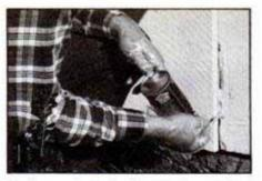
To close gaping holes, foam sealant worked the best, but it was hard to control in narrow confines. To seal smaller leaks at windows and doors, we used caulk in a gun.
