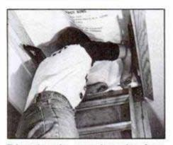
This attic stairs cover (mounting frame included) zippers shut to seal off the attic opening. The cover prevents warm air from leaking out of the house into the attic.
