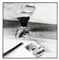
Fit the lock into the front of the box. I removed most of the wood with a chisel, then used a high-speed hand grinder in the finishing stages. You may prefer to do this job before you start assembling the desk.
