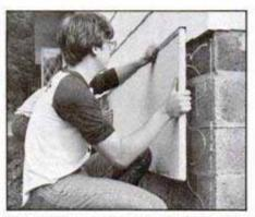
Foundation insulation is applied to reduce heat loss through the block. Since the insulation was thicker than the siding, we added protective top trim.
