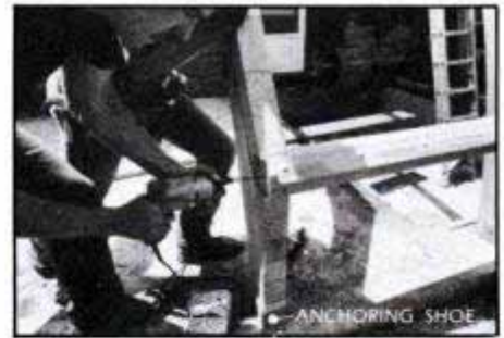
Beam feet rest in metal shoes anchored to slab with lag screws in lead anchors. Cross braces are fastened with screws.
