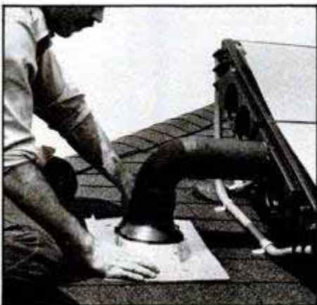
Permanent installation of the roof duct is through a roof flange. Latter is installed with upper edge under shingles. All edges are then sealed with caulk.
