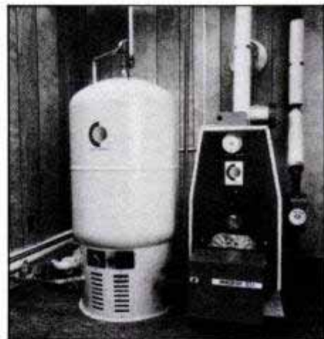
Circle Combustion's compact boiler and water heater use heat-purging systems.
