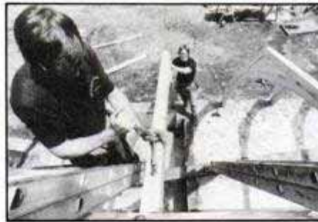
Preformed beam tops are fastened to the ledger with lag screws. The recess in the slab here will accommodate a hot tub.
