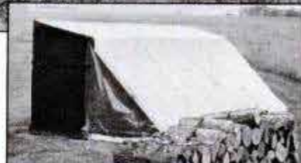
Logs being seasoned rest on 4x4 skids in 2x4-framed, plywood-sheathed dryer (above). Interior is flat black and top exterior is white. The front is covered by clear plastic (right). Materials cost $80.
