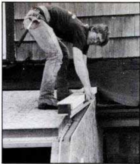
End filler component joins roof to end-wall. Topside, it is nailed to beam. It joins sidewalls with splines and nails.
