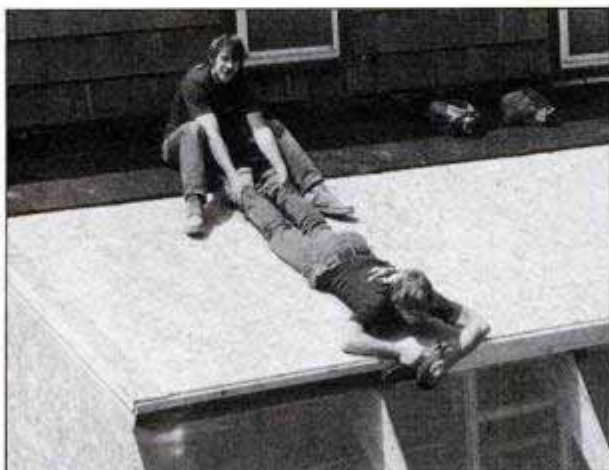
Adding a solar room: A job for circus aerialists?
