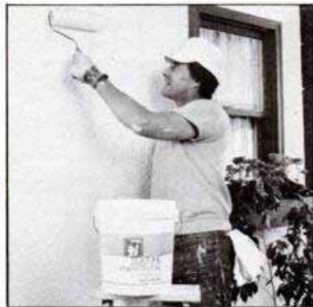
Mask wall repairs while painting the wall with Textone Ready-Mixed Textures.
