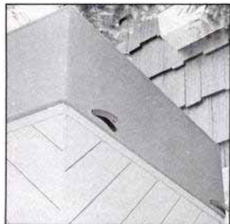
Drain tubes inserted in holes bored in the rear of planter direct water away from the shed to eliminate water stains.
