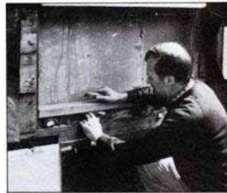
Use utility knife to cut back insulation.
