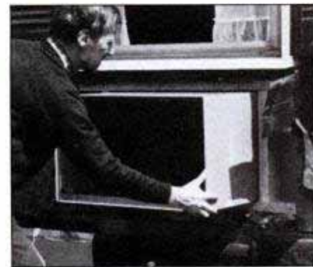
Check fit of case, then finish nailing.
