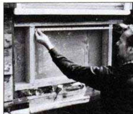
Check framing dimensions for the case.
