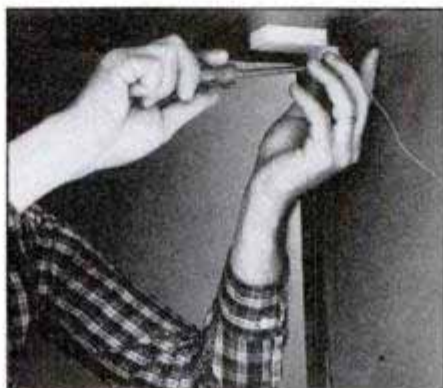
Screw case to frame after positioning with slight pitch to outside for drainage.
