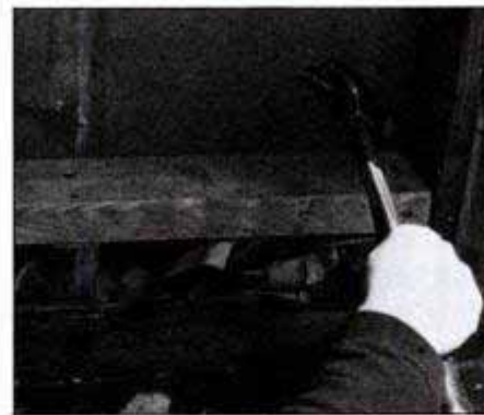
Toenail sill, here, and header into place.
