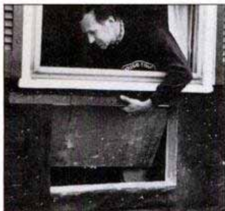
Cut out wallboard flush with the frame.
