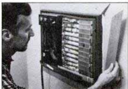
Before installing the molding, caulk between wallboard and case to cut drafts.
