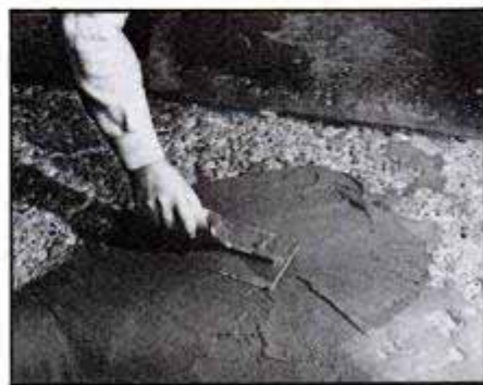
The patching mix used consists of 1 part portland cement, 2½ parts sand and enough water to allow paste to hold its shape. Apply with a smooth trowel.
