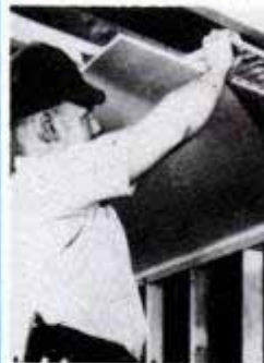
See how to install ceiling panels by several methods.
