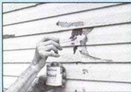
Step 2: Use thin, even coat of glue on any bare spots. Overlap the paint edges.
