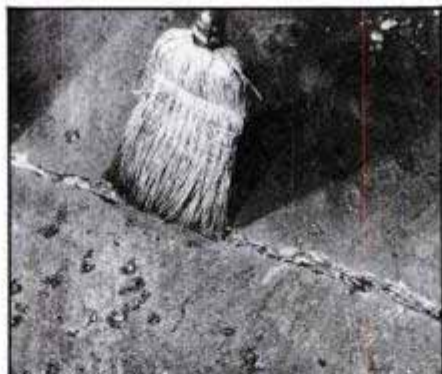
Clean the crack thoroughly to remove any particles that can weaken the bond.
