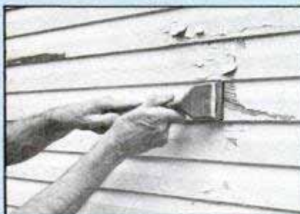
Step 1: Scrape off all the peeling paint; feather the remaining edges smooth.
