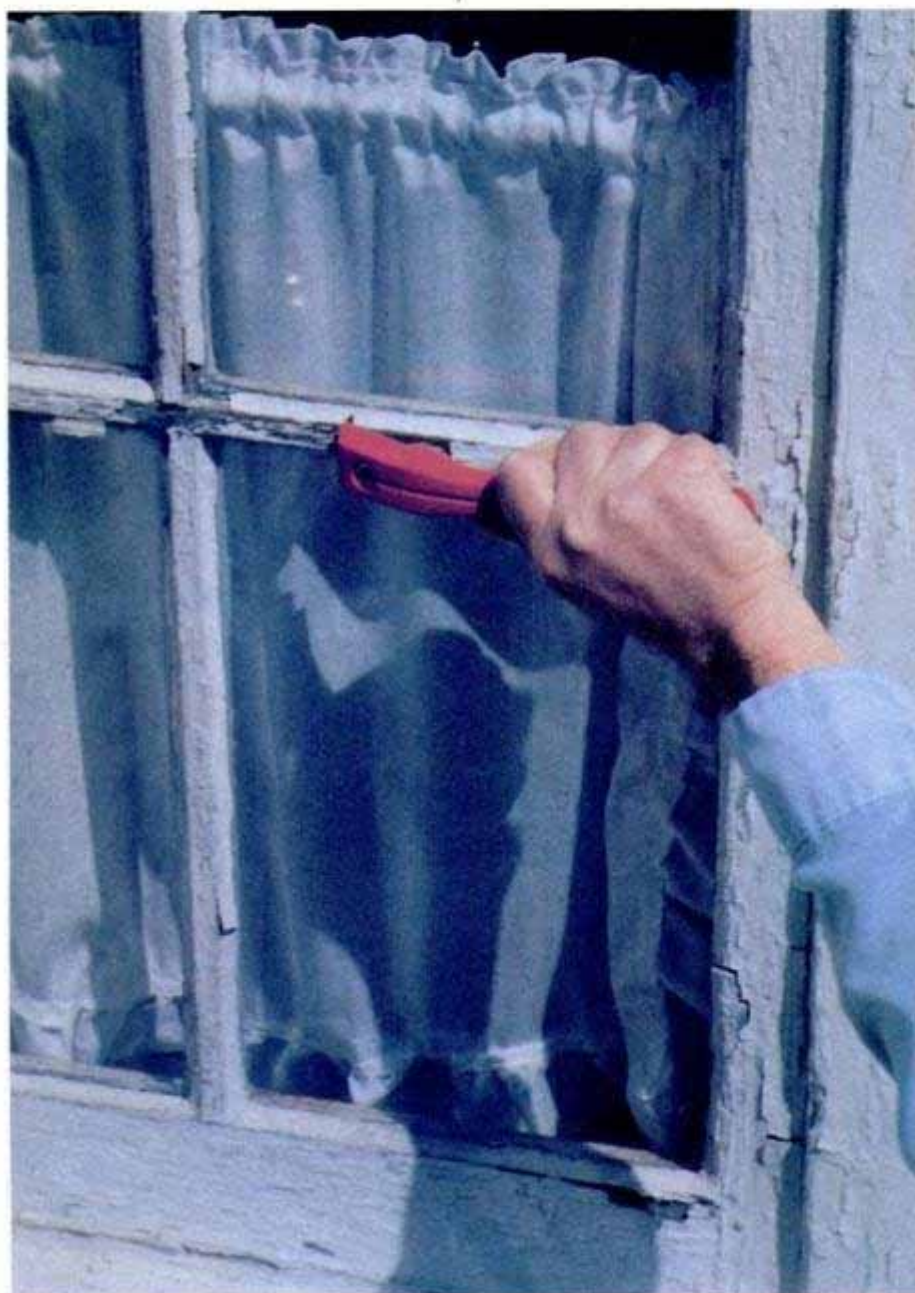
The majority of paint problems are caused by moisture. Originating inside the house, moisture absorbed by this window frame has lifted the paint. To correct the problem and save hours of scraping and repainting, venting is needed.
