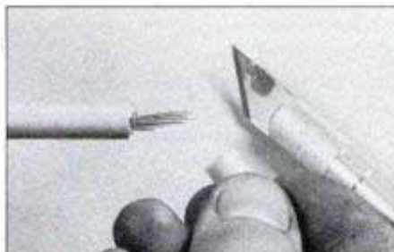
With a sharp knife, slice off about a half inch of insulation. Don't cut any strands of wire while trimming.
