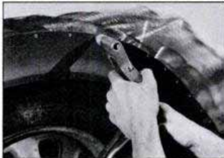
If the replacement panel is aligned properly, drill holes every 4 in. around the perimeter and install the rivets.
