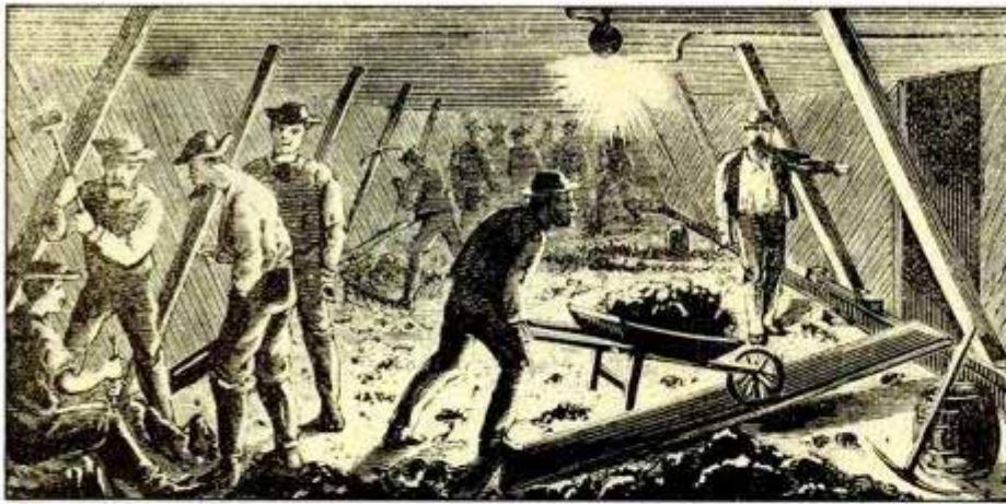
Inside the work chambers under the caisson, crews of 30 to 40 men broke up riverbed around cutting edges to allow caisson and bridge tower to settle down to the bedrock.
