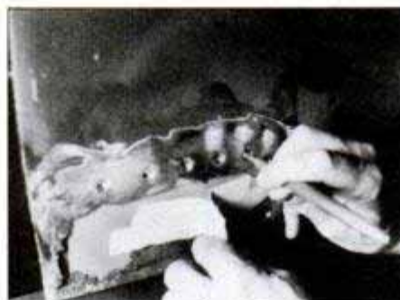
Insert the metal patch and mark it for the holes with a felt marker. Hold the patch steady while you're doing this.
