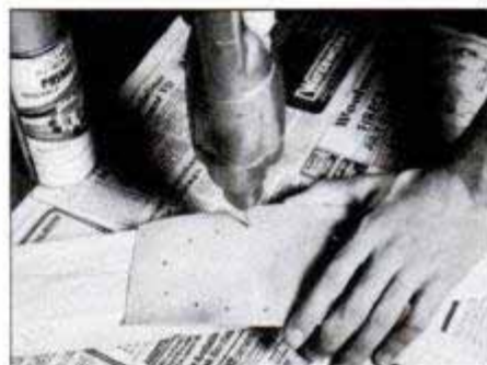
Drill \frac{3}{32} -in. holes in the marks. Use a low speed and don't let the drill bit wander on the metal patch. Keep the handle on.
