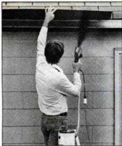
Use hardboard or cardboard strip for a handheld shield to protect adjacent surfaces, such as roof shingles, from overspray.
