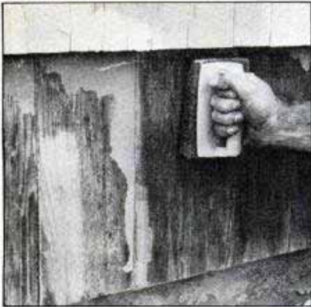
A special scrubber tool is useful for cleaning and smoothing rough surfaces.
