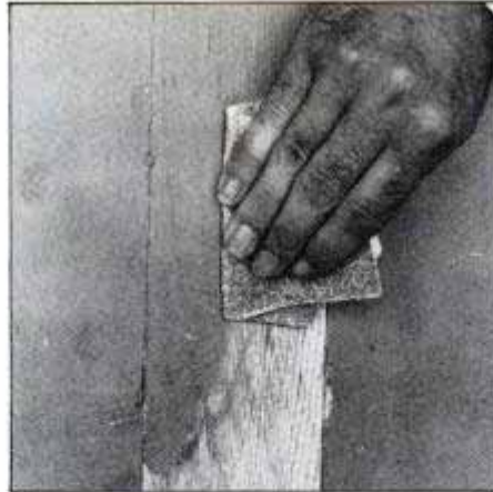
For a smooth finish use 100-grit sandpaper to feather all sound paint edges.
