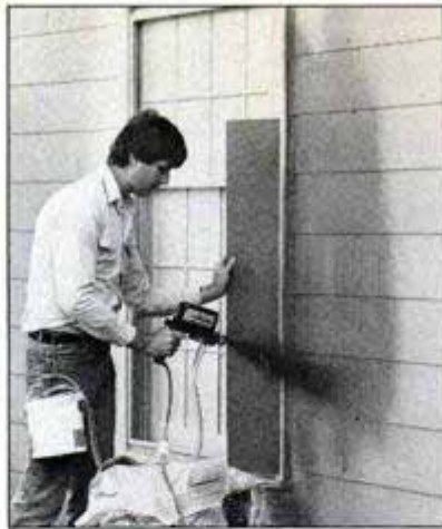
Use shield to mask trim from the siding color. Here, casing face is left partly exposed for thorough coverage at siding-casing angle.
