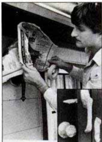
Mask fixtures, doorknobs and latches with paper or plastic. Tape lamp base carefully for even contrast line.
