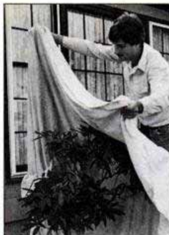
Cover plants near the house with dropcloths. Cut or tie back all foliage that brushes against the siding.
