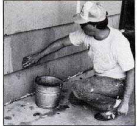
Remove mildew and chalking stains by washing with a solution of trisodium phosphate, detergent, bleach and water.
