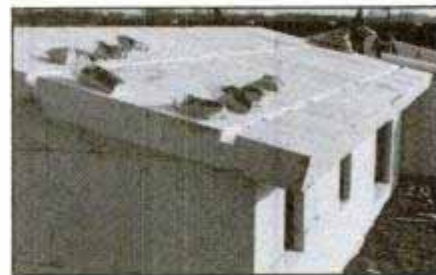
The polystyrene roof was tested with a load of 7 tons before it was installed.
