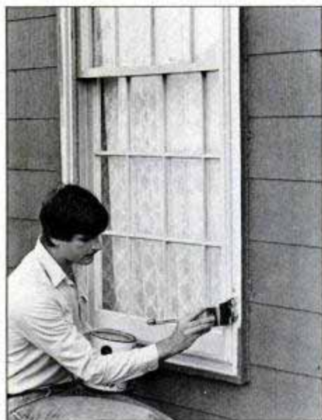
Touch up the oversprayed areas on the window casings and other trim with a brush when paint is dry to the touch.
