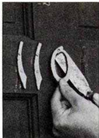
Before spraying, remove all nameplates, screens, storm sash and other fixtures that are difficult to mask.
