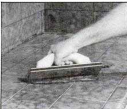
12 Allow adhesive to set at least 24 hours before grouting. Use a rubber-faced trowel or squeegee to press grout into joints and remove excess from tile.
