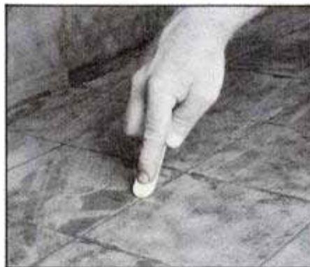
13 Use a tongue depressor or similar tool to compact grout and remove buildup at the edges. This technique is referred to as "striking the joints."
