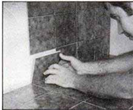
10 Grout joints on backsplash should align with those of countertop. If a course needs to be cut to fit under hanging cabinets, it should be top course.
