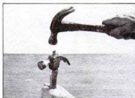
7 To ensure a completely tight fit, the metal wedge is then hammered fully home. Take care not to drive in the wedge until it is properly positioned.
