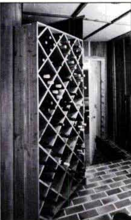
Wine rack acts as door to mechanicals room. Bottles disguise the room, while the open shelves allow free air circulation for efficient operation of the heat pump.
