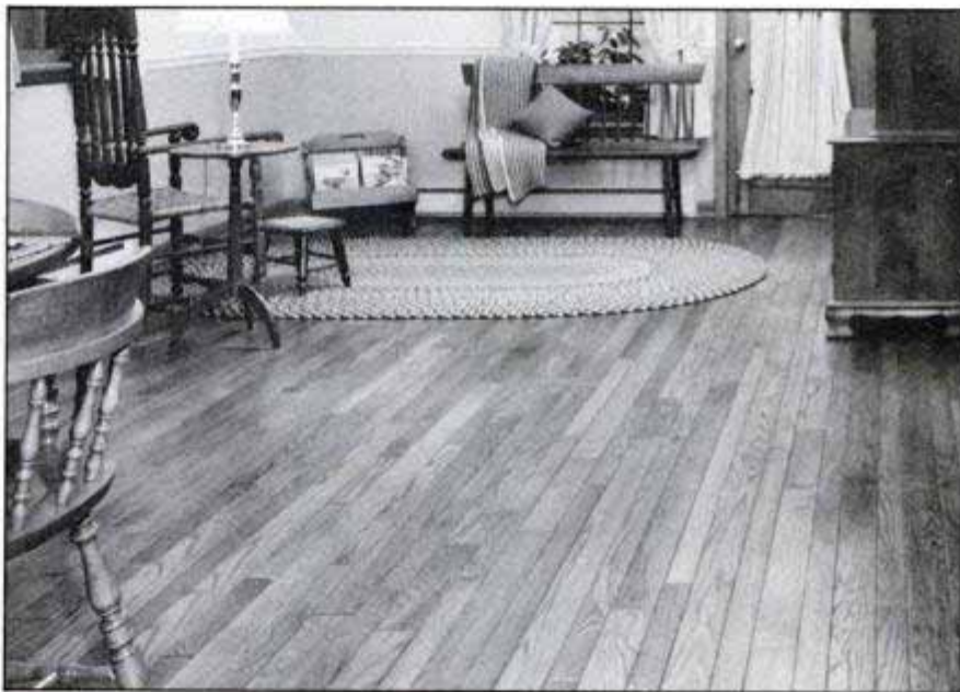
We covered an old resilient tile floor with prefinished oak strips to give our family room new warmth. Installation is easy, requiring use of only a few special tools.
