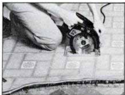
To prepare for the installation, we first removed the base shoe, baseboard molding and the covers of the baseboard heating units from the perimeter of the room (above, left). We used a circular saw, set shallow, to cut a straight line across the room, squaring off a curved seam where two floor coverings met previously (above, right). The new oak strips run across the void, bridging the slight depression.
